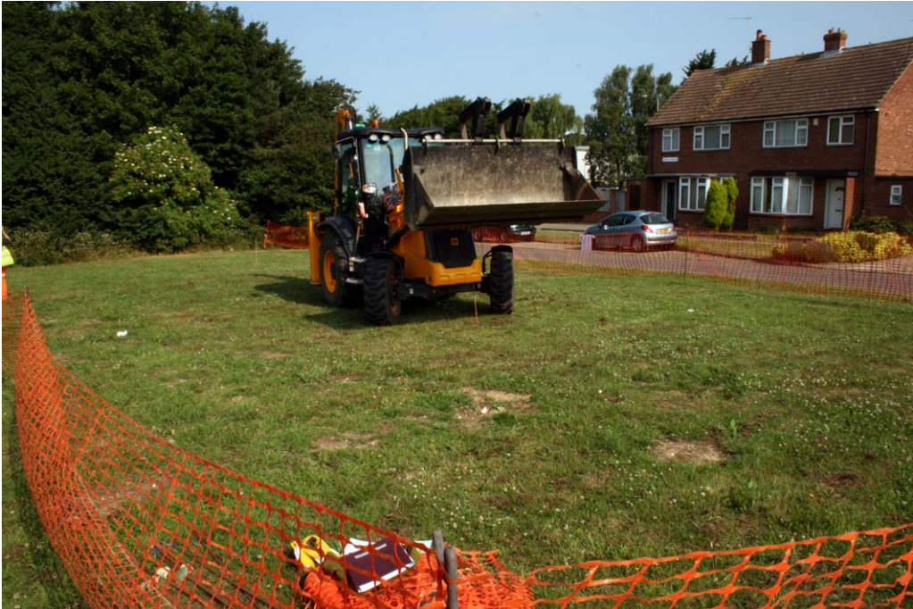
Plate 1. The site looking north-west
