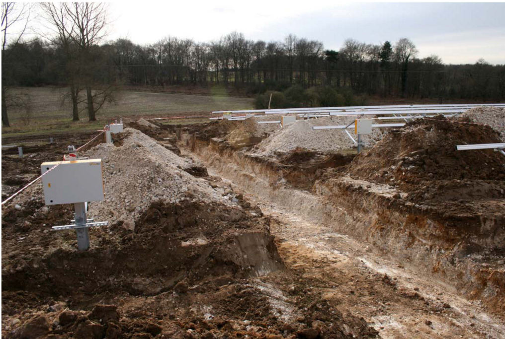
Plate 1. The site looking south
