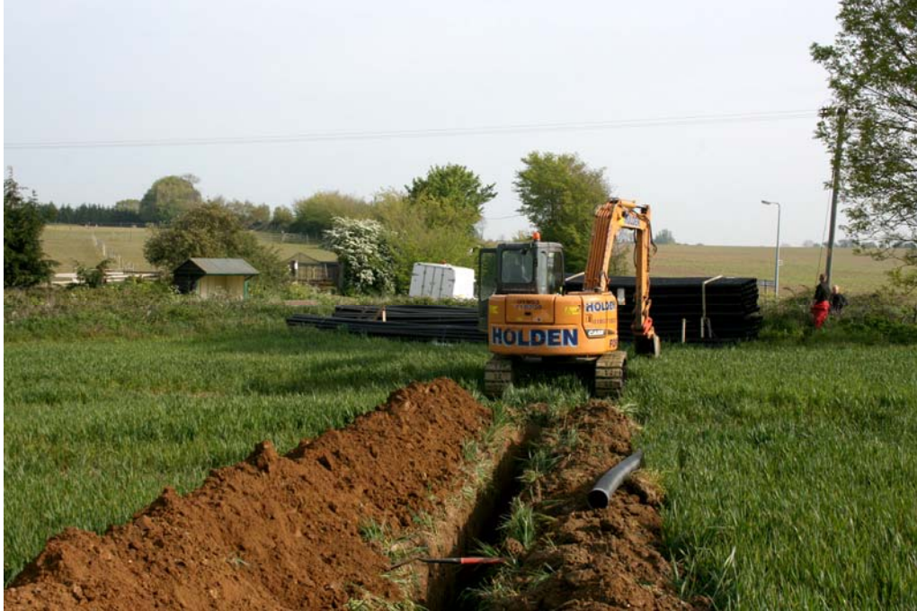
Plate 2. Cable trench looking south
