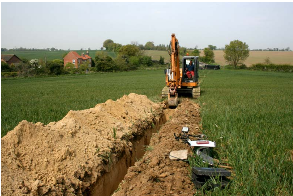
Plate 3. Cable trench looking north
