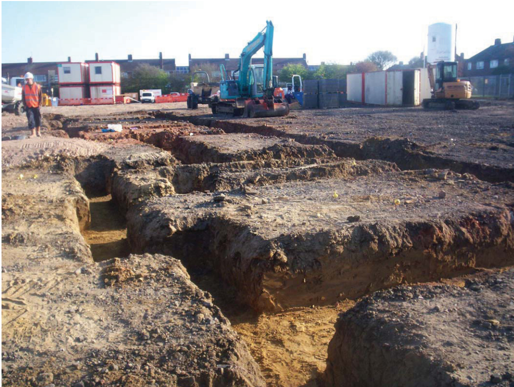
Plate 2. Excavation of the foundations facing north
