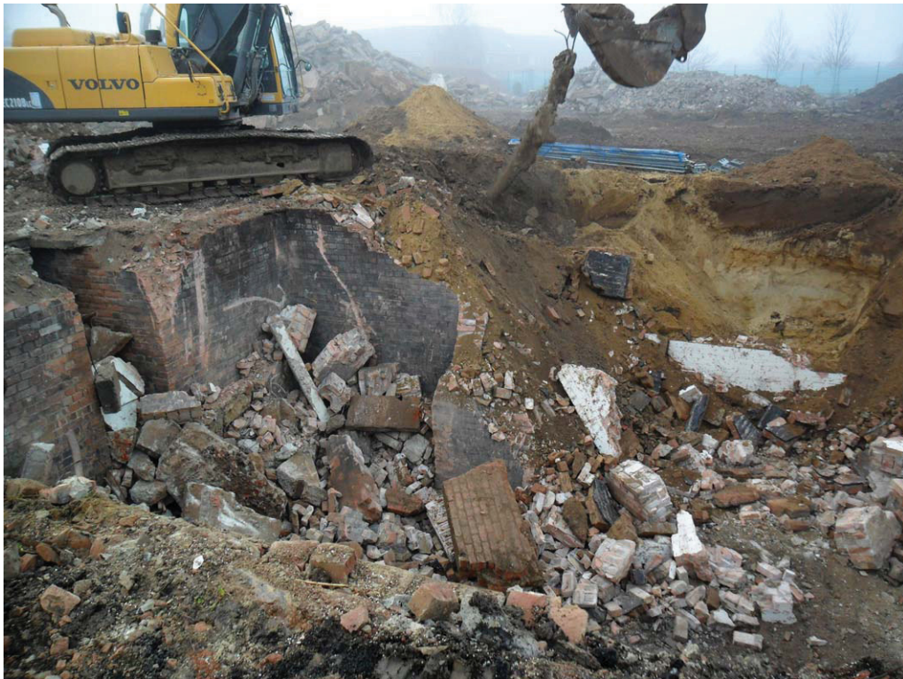
Plate 1. Demolition in progress
