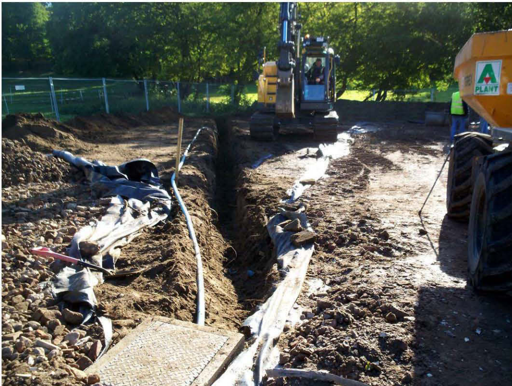
Plate 2. The water pipe trench, facing north-east
