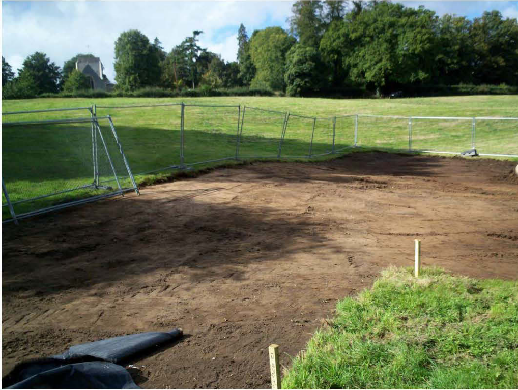
Plate 1. Topsoil strip facing west
