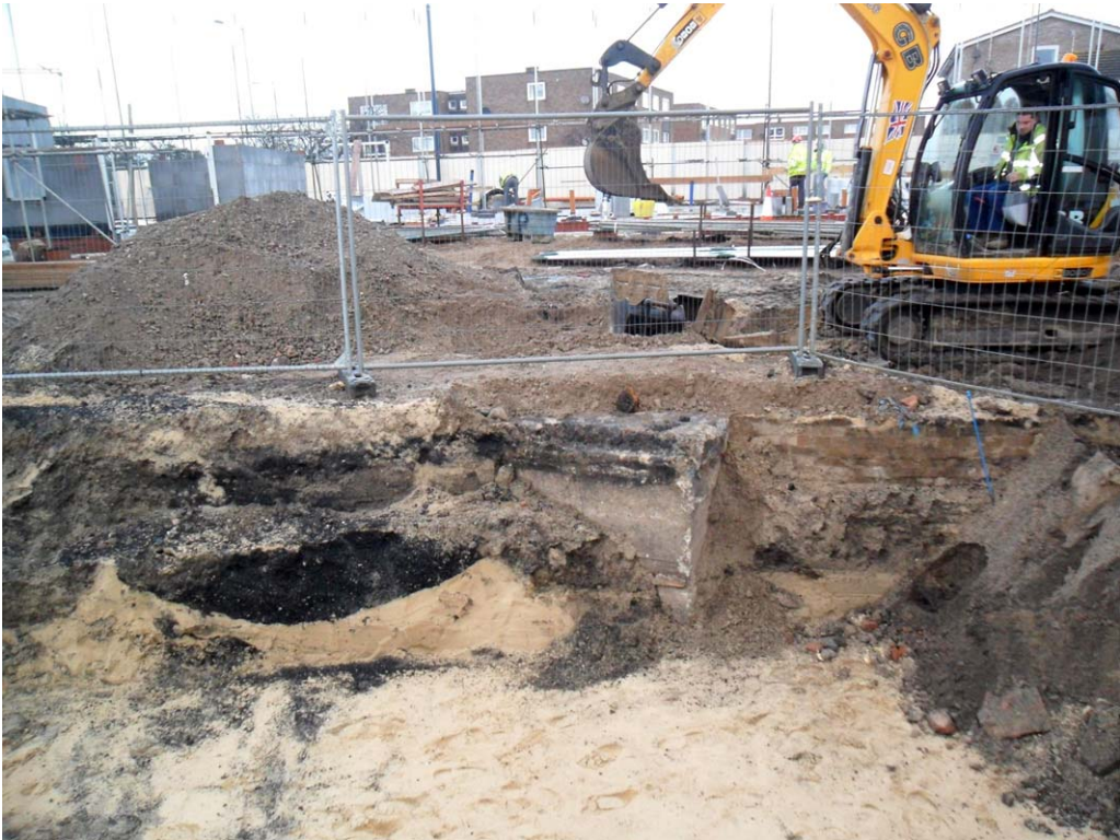
Plate 4. Opposite side of the turntable pit, facing north
