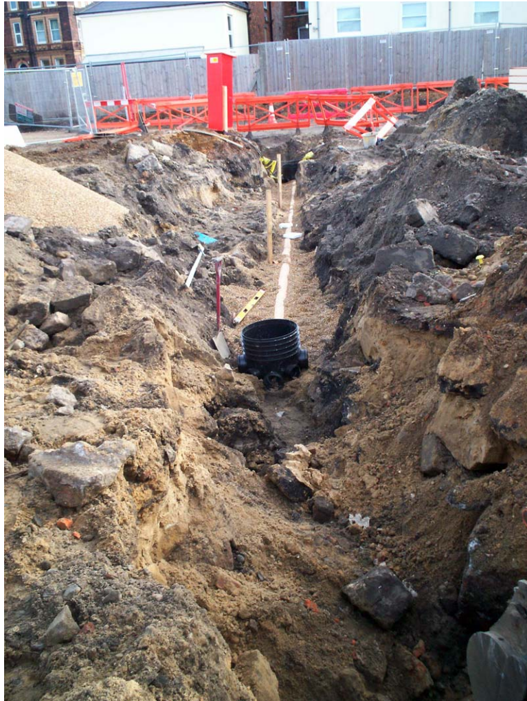
Plate 2. Sewer trench through the site of the turntable pit, facing east
