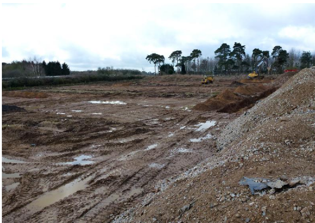
Plate 1. The evaluation site, looking southwest
