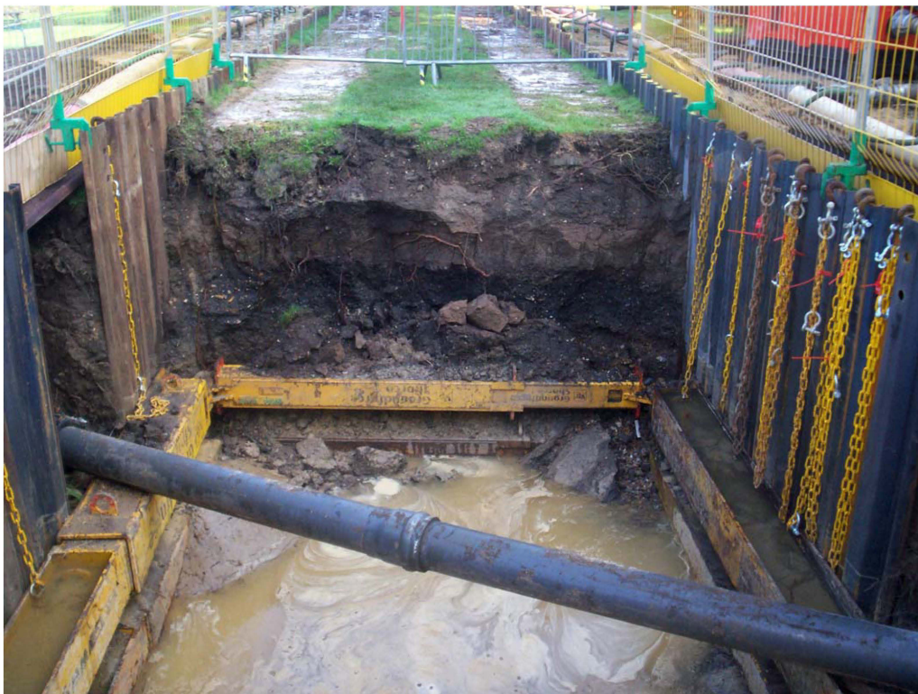
Plate 1. The southern end of the trench, facing north
