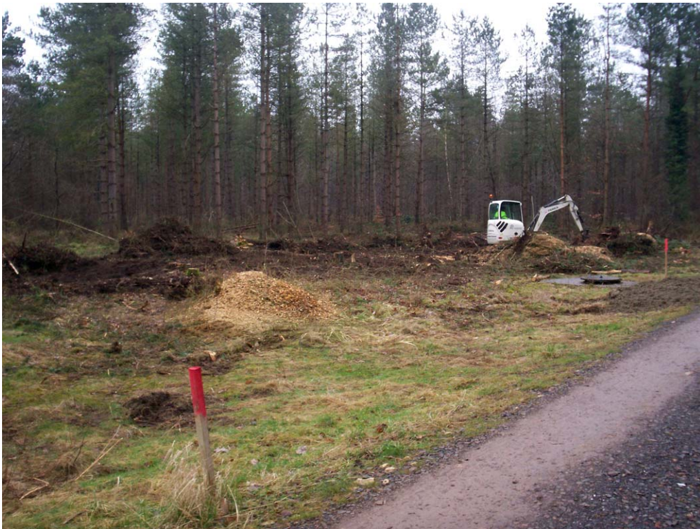
Plate 1. Borehole G destumping facing north-east
