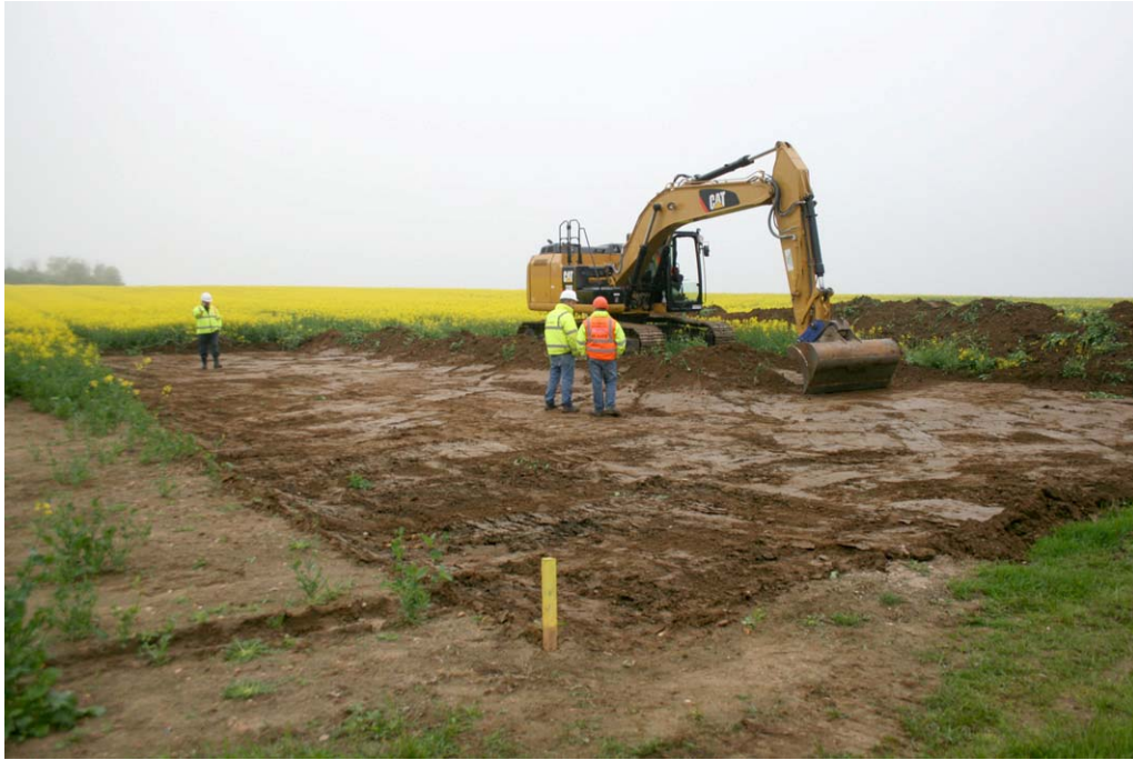
Plate 1. Leziate Drove Pumping Station, site stripping
