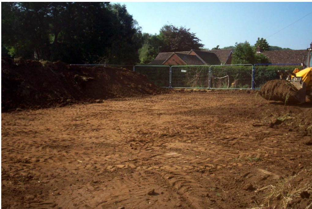
Plate 2. Fen Lane Pumping Station, site stripping
