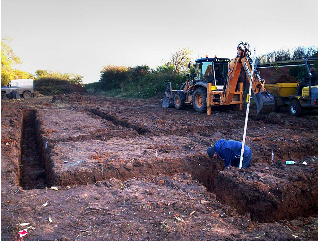
Plate 1. Excavation of foundation trenches, looking southeast
