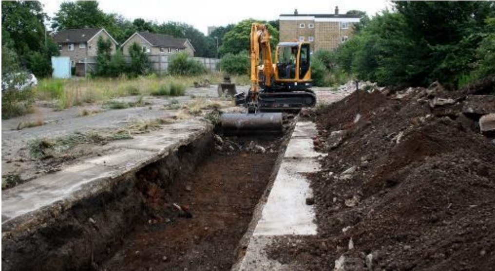
Plate 1. Machining Trench 3, looking south
