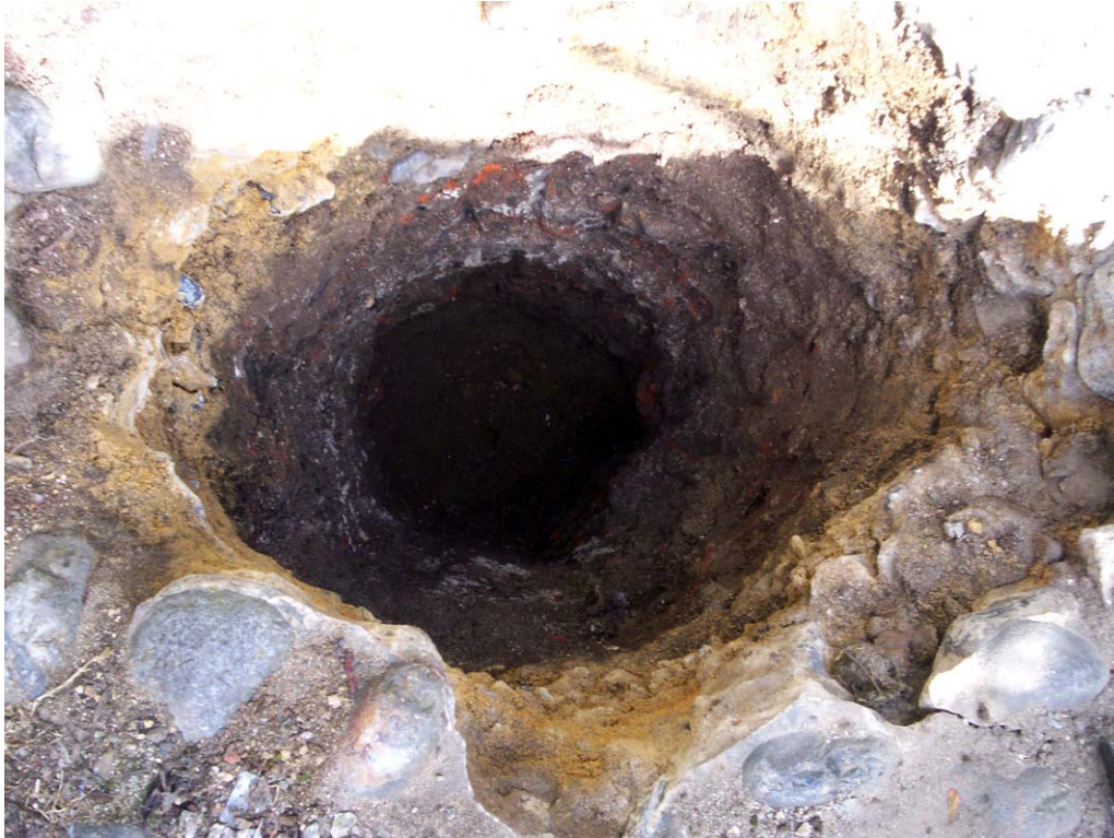
Plate 2. The earth rod excavation, from above
