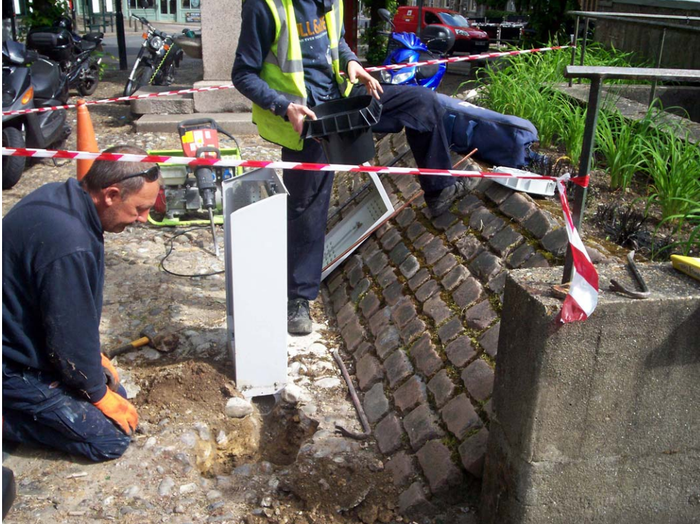
Plate 1. The excavation, facing north
