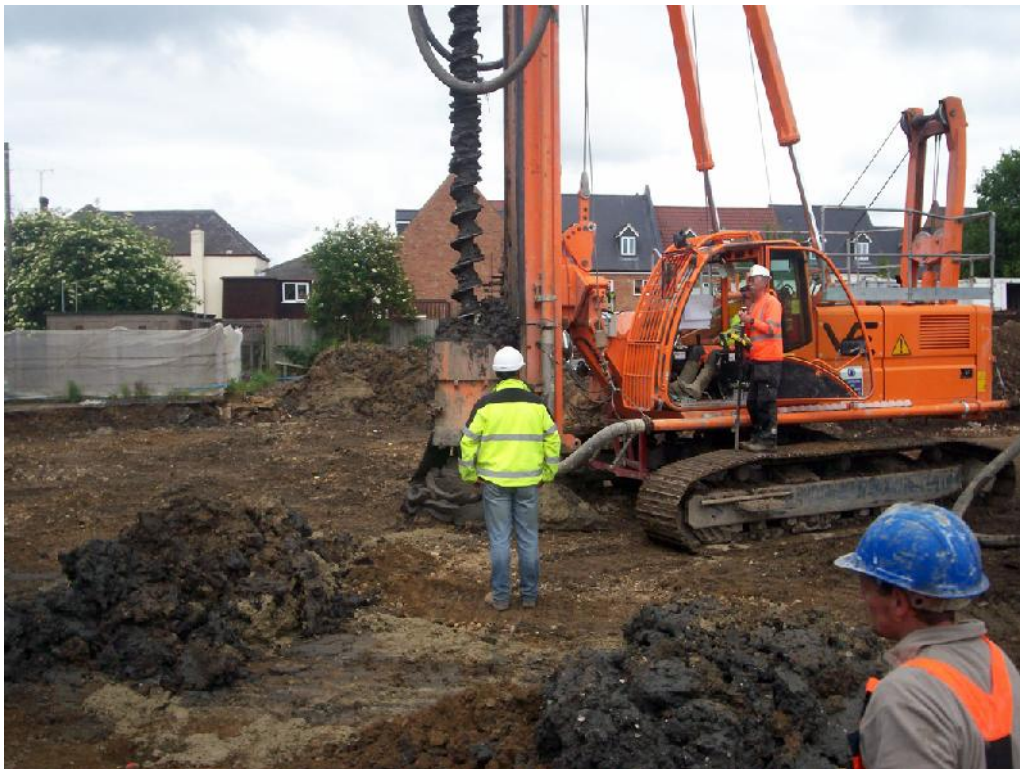
Plate 1. Piling in the northwestern corner of the site
