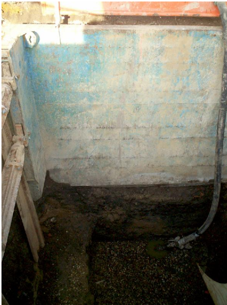
Plate 2. Manhole 2 facing northwest
