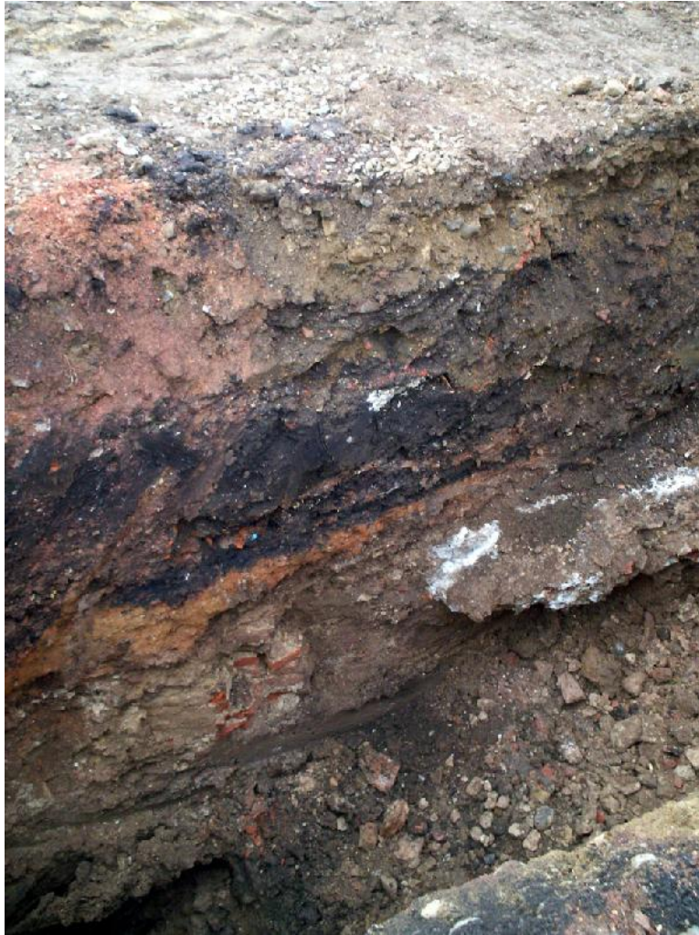
Plate 5. Wall {66} facing southwest (the concrete to the right is a foundation of the former cinema)
