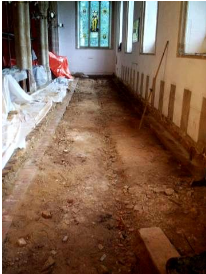
Plate 1. The south aisle before excavation
