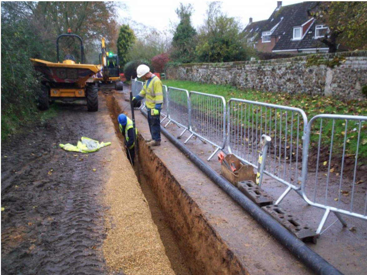
Plate 1. The open trench facing north
