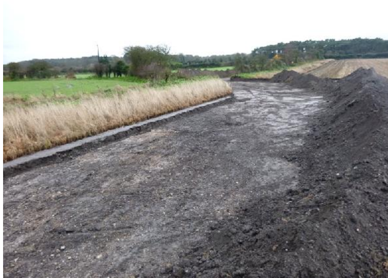
Plate 4: Deposit 21 , the gravelly material in the centre, facing southwest
