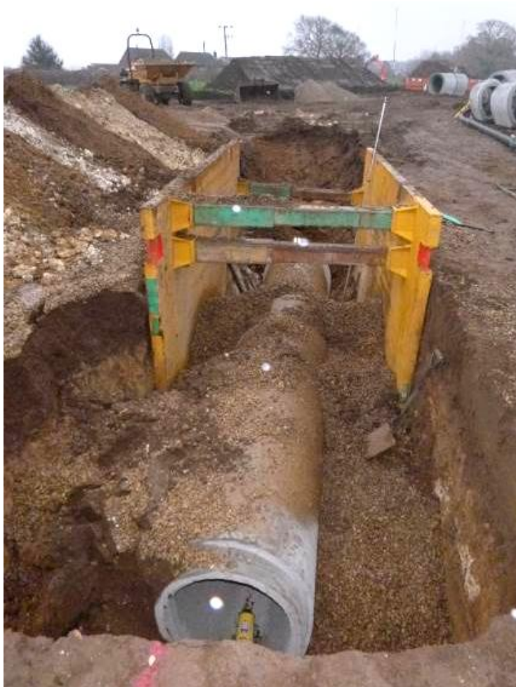
Plate 3. West end of the pipe trench facing east
