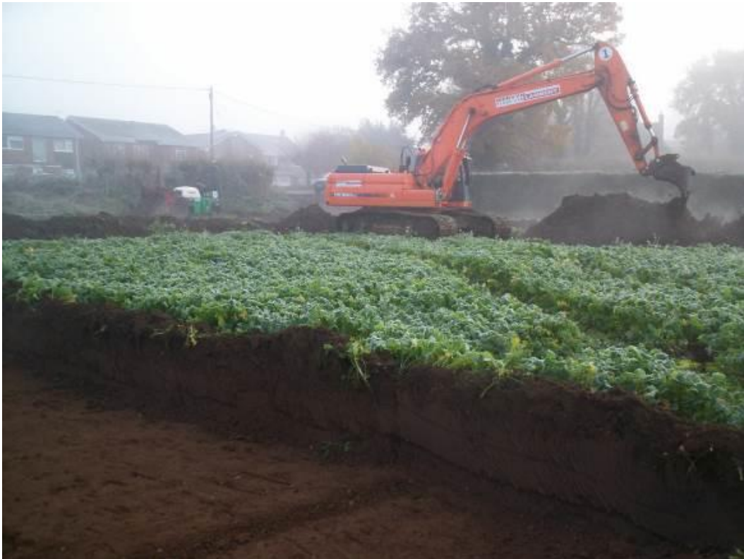
Plate 1. Compound area topsoil strip, facing east
