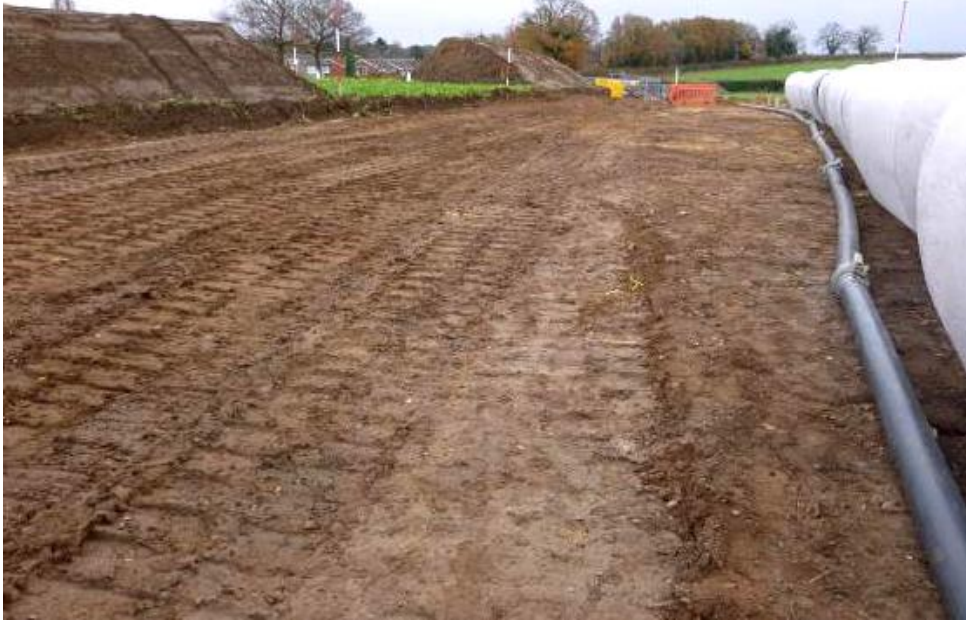
Plate 2. Stripped pipe trench easement, facing east
