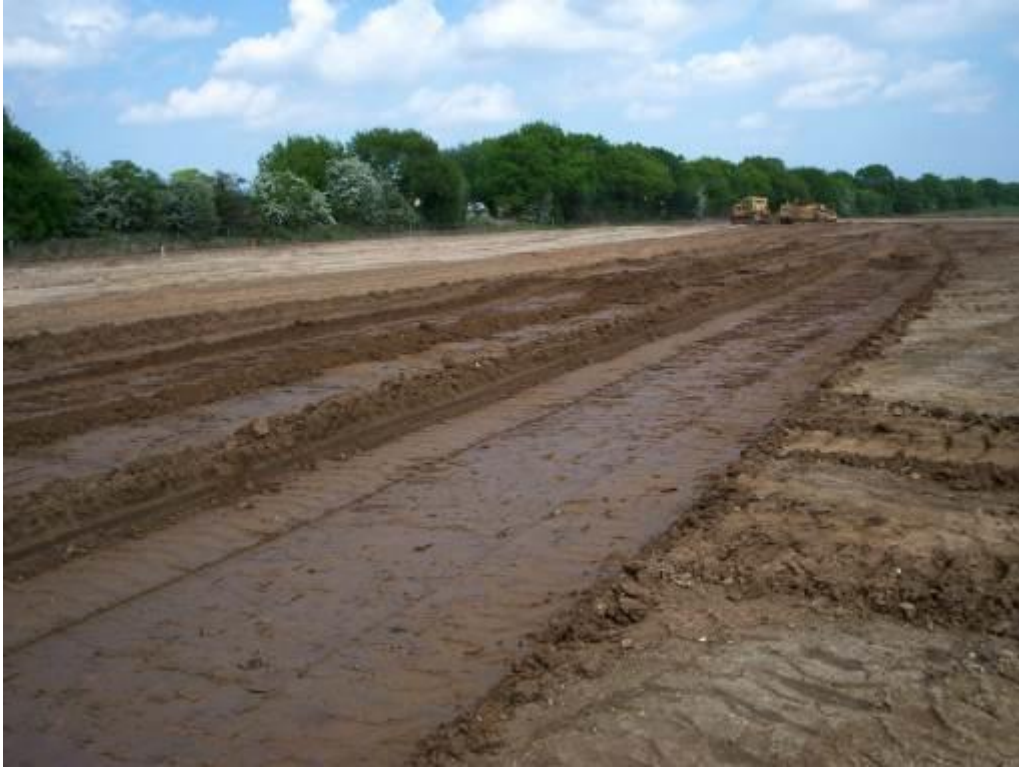
Plate 1. Grading the football pitches facing northeast
