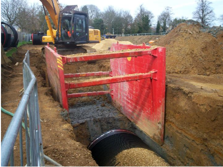
Plate 1: Pipe trench looking northwest
