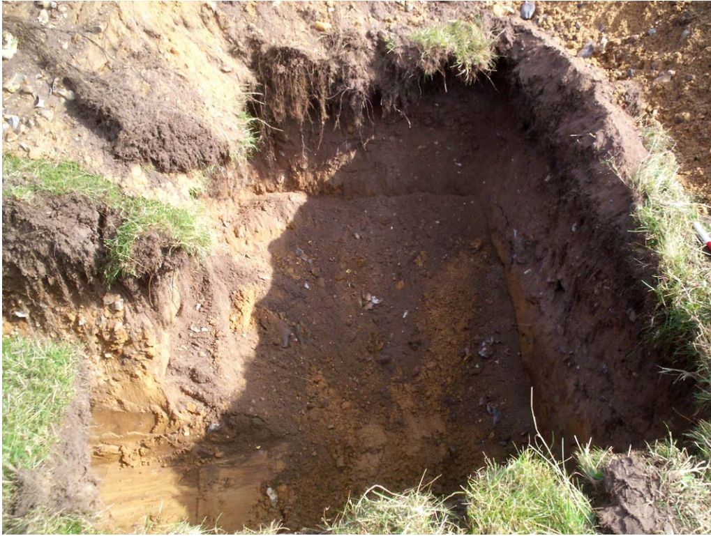
Plate 3. Directional Drill Pit 1, facing northeast
