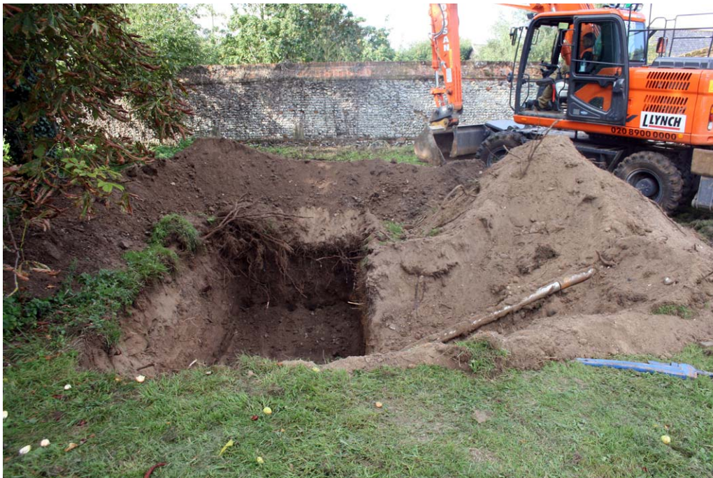
Plate 2. Directional Drill Pit 2, facing northwest
