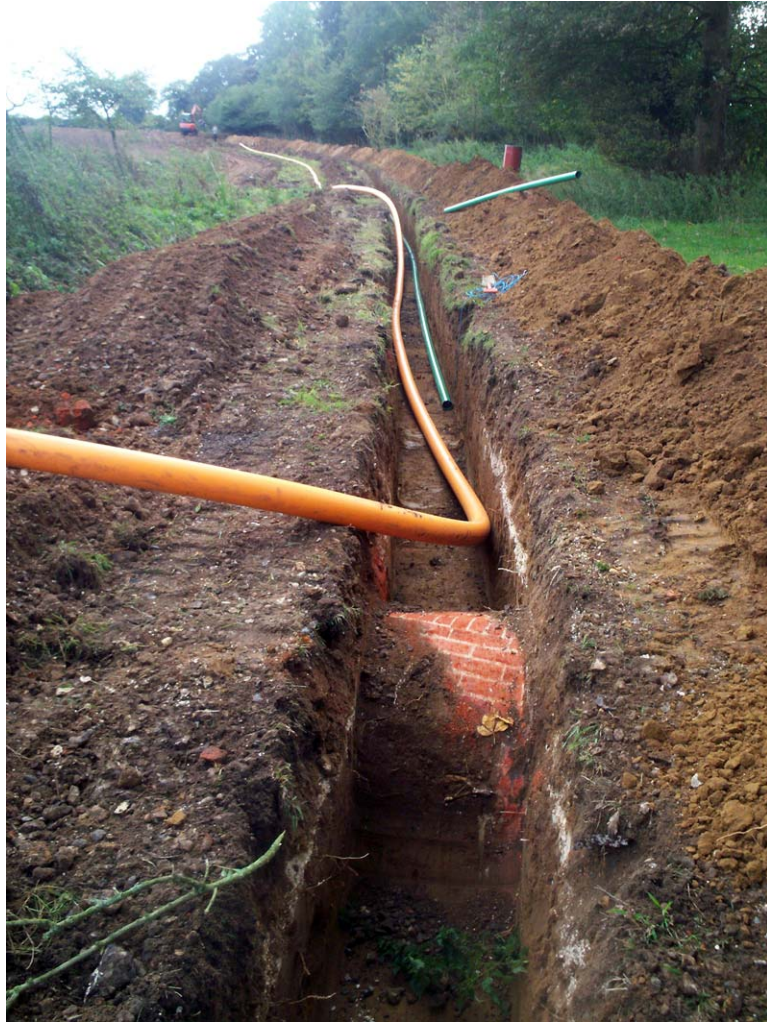
Plate 6. Culvert {10} facing south
