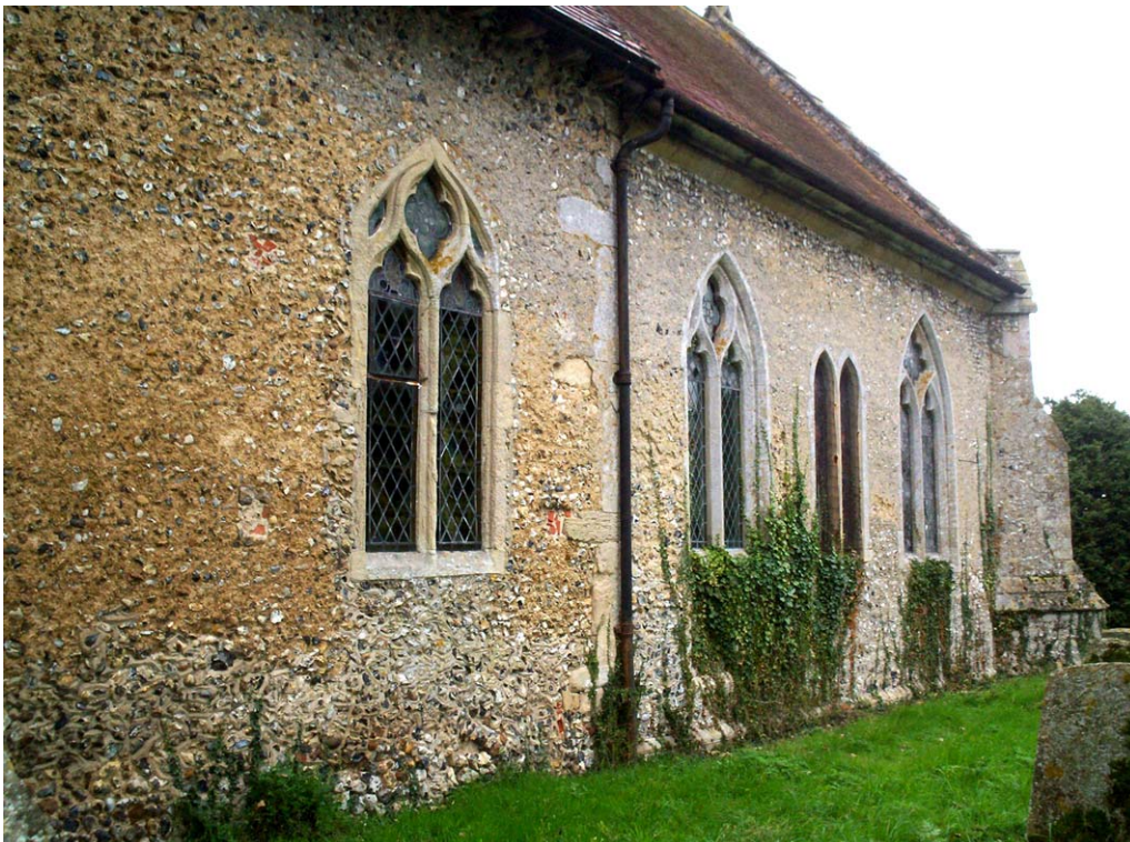
Plate 1. 'Long-and-short' quoins at the east end of the nave, facing northeast
