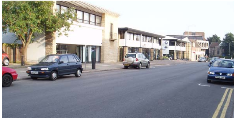
Plate 1. The East Site, from the north, looking towards the Ber Street frontage
