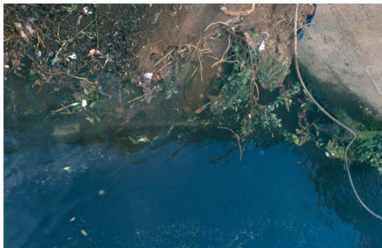
Plate 2. Cleared bank showing in situ wooden revetment, looking south-west
