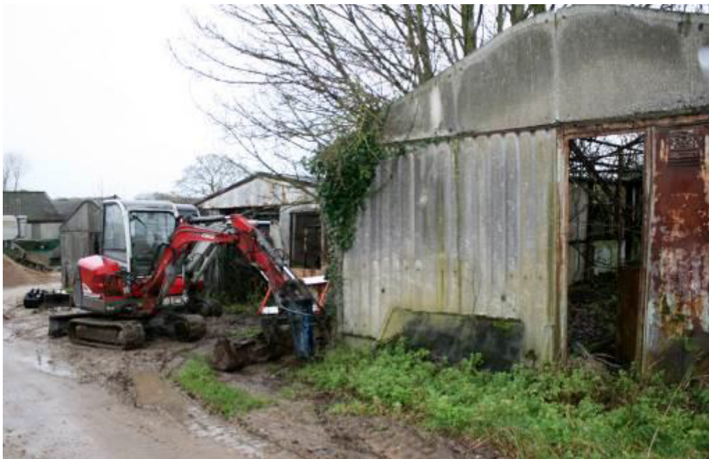
Plate 5. Sheds and barns on the site, looking southeast
