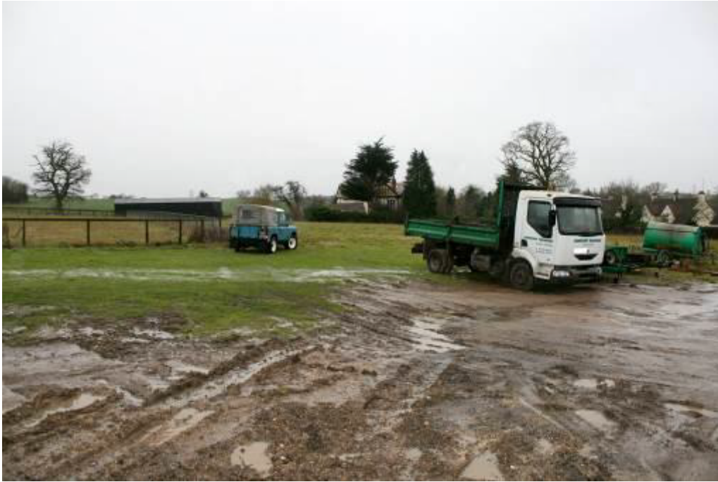
Plate 10. View to the south from the site
