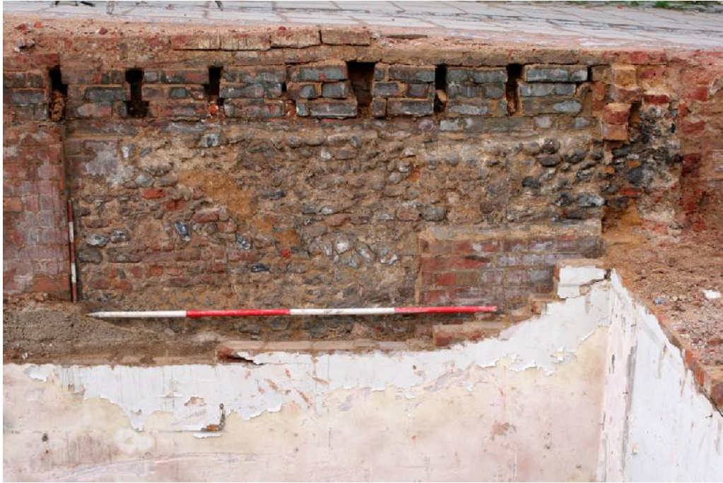
Plate 8. South-facing elevation of wall 25
