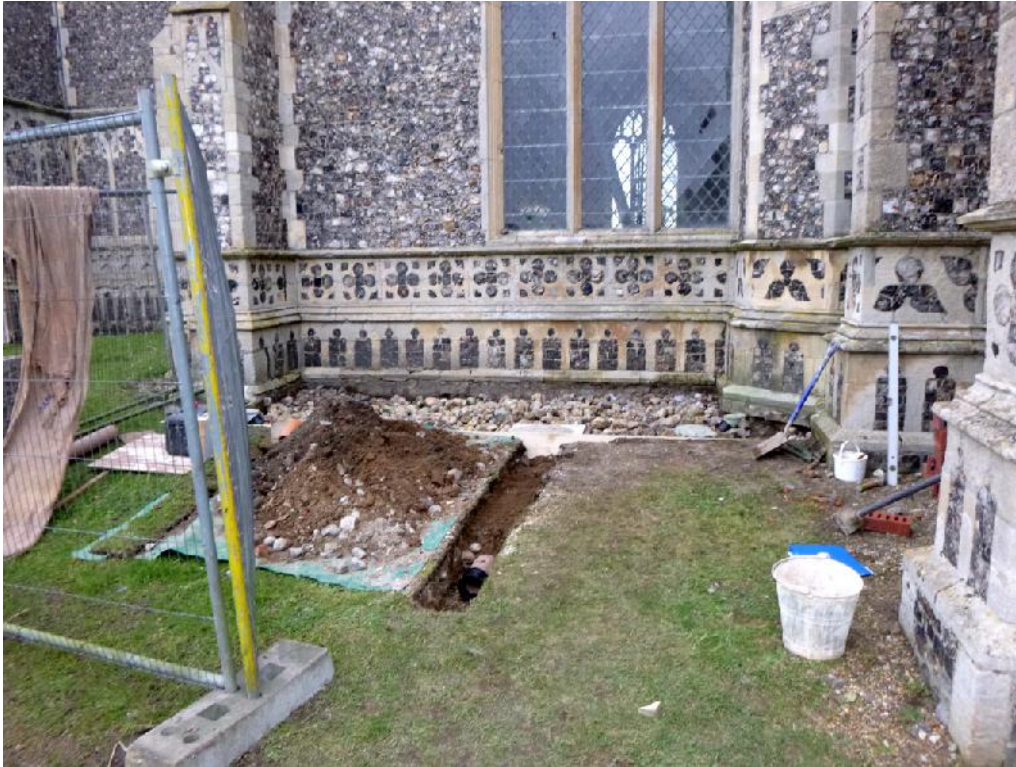
Plate 1. The rainwater catch-pit, looking north
