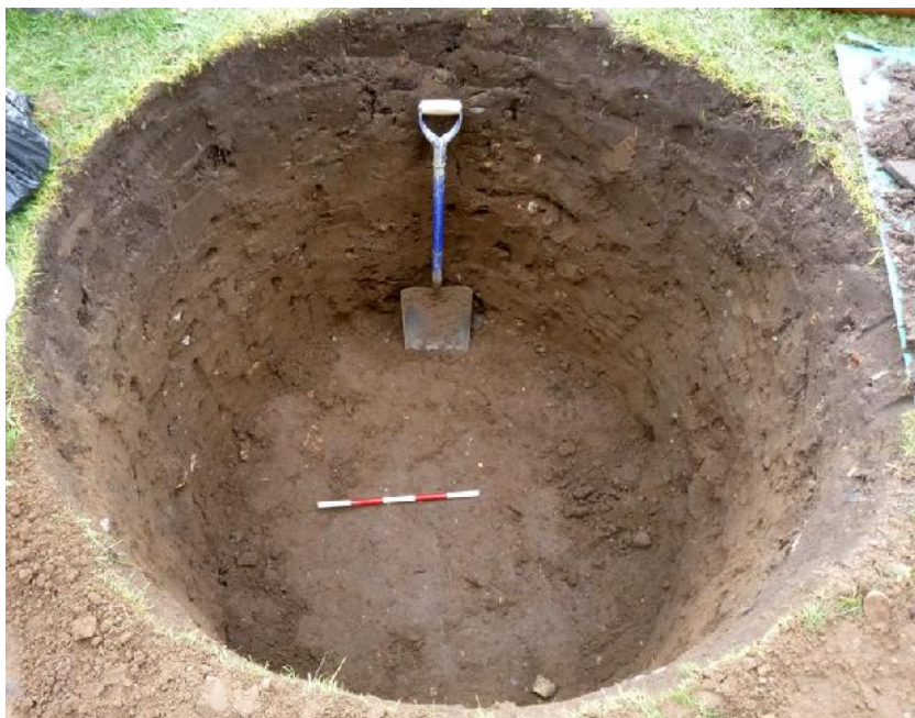
Plate 3. The soak-away under excavation, looking south
