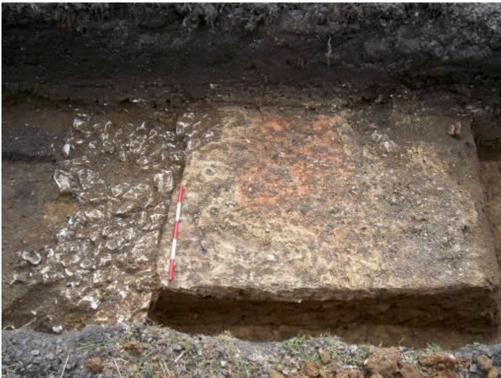
Plate 5. Period 2 foundation 28a and floors 07a and 08a (Structure 23 ), looking south
