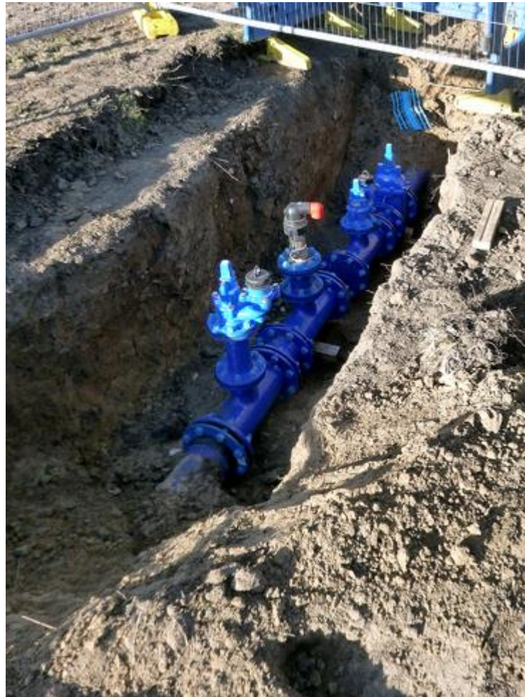
Plate 1. The Field 1/Fakenham Road trench, facing north
