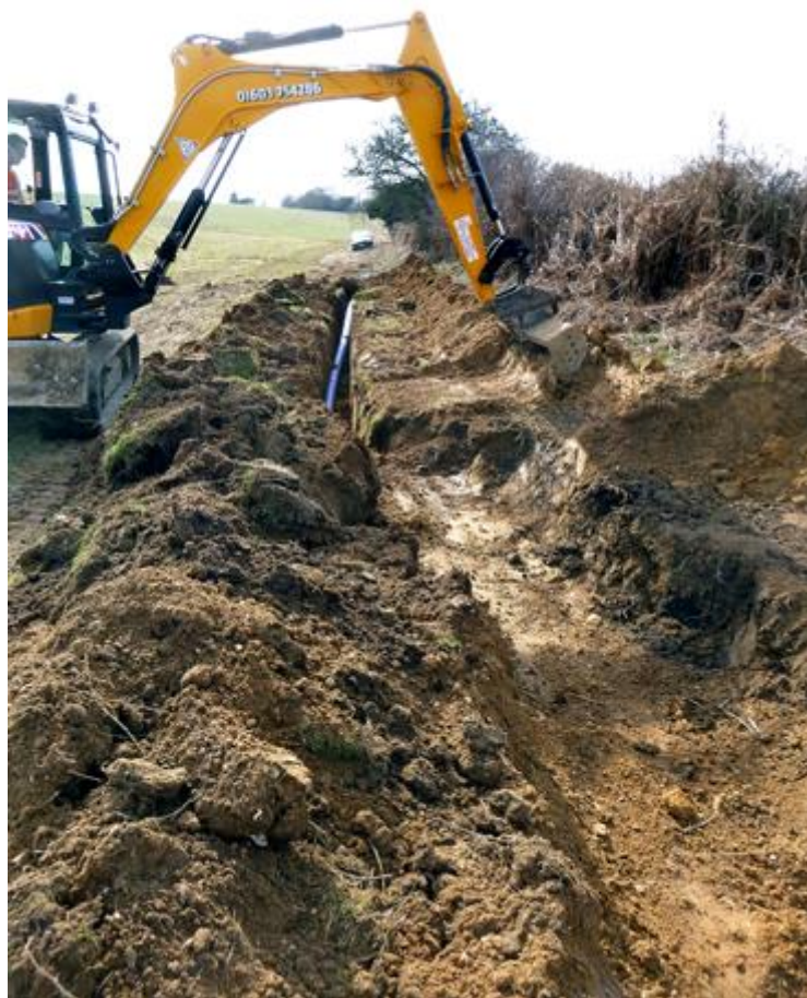
Plate 3. The open-cut trench in Field 1, facing south-southwest
