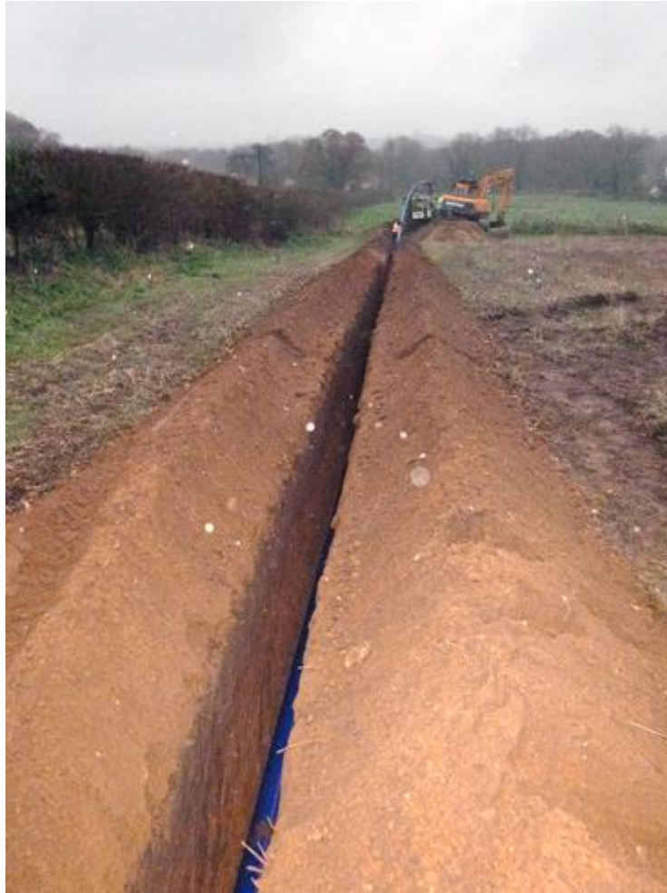
Plate 5. The mechanical trencher in Field 3, facing south
