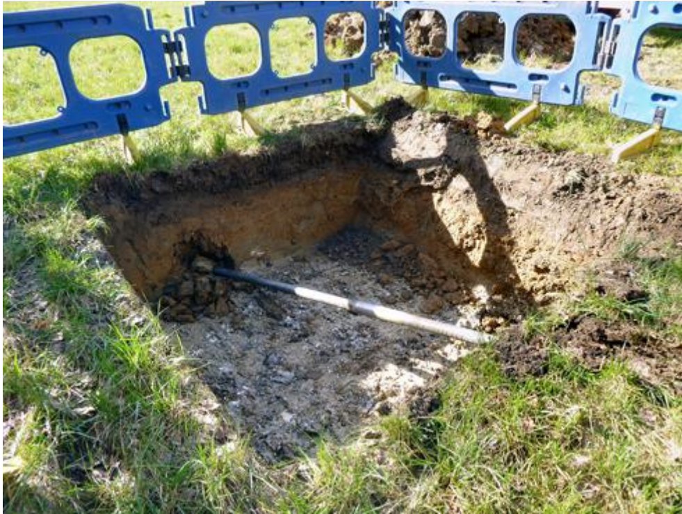
Plate 2. The Field 1 directional-drill pit, facing west
