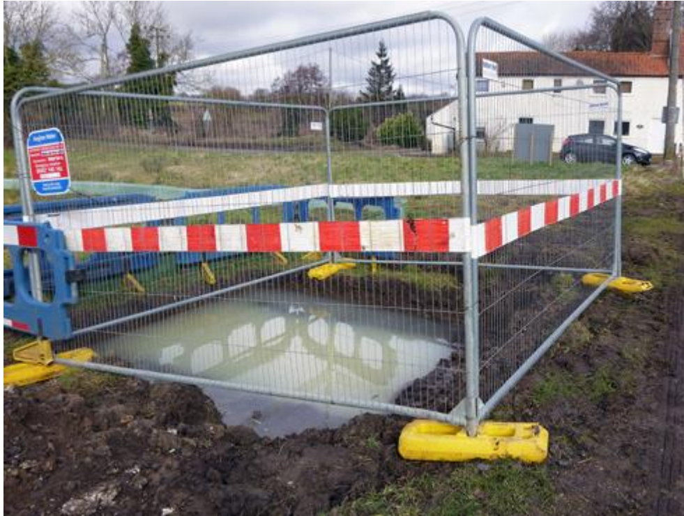
Plate 9. Directional-drill pit in Field 11, facing north
