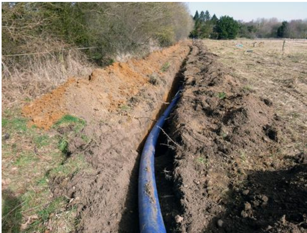
Plate 4. The open-cut trench in Field 2, facing north-northeast
