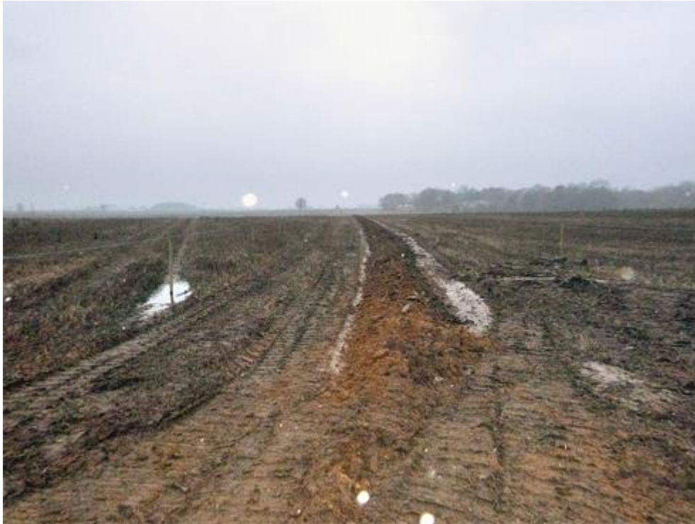
Plate 6. Field 5 after backfilling, facing north
