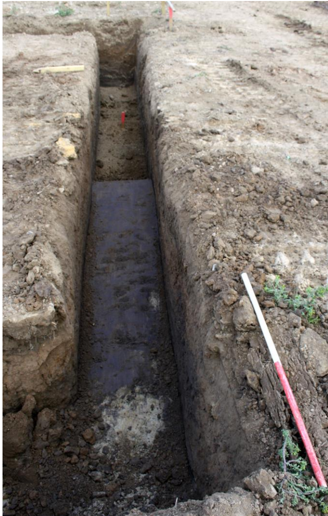
Plate 11. Plot 4; palaeochannel 08 in foundation cut
