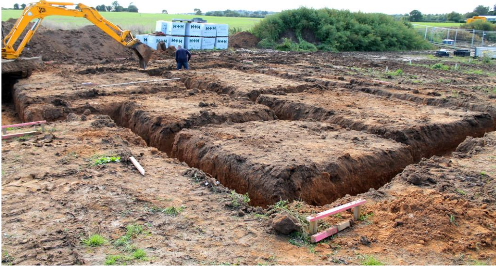
Plate 15. Plot 8; general view facing southwest
