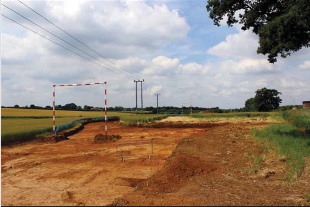
Plate 1. Area A, looking southwest
