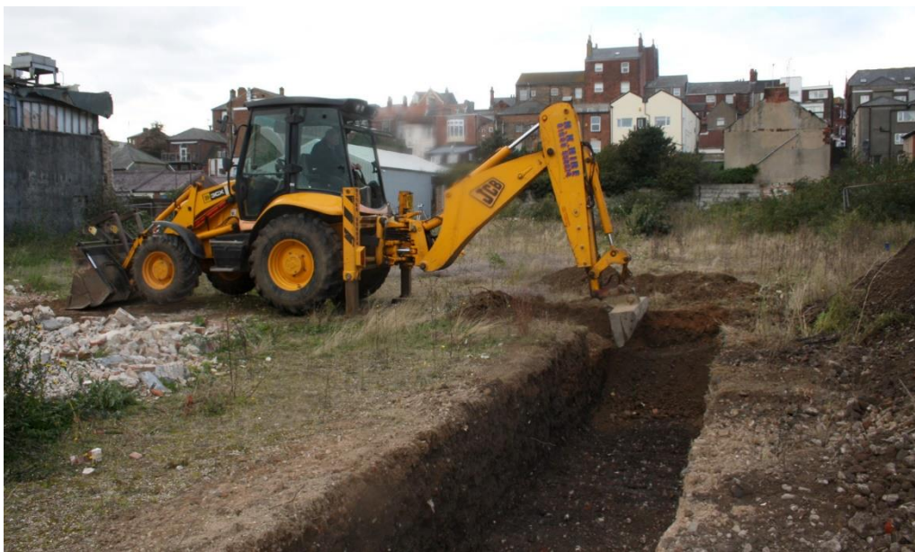
Plate 1. Mechanical excavation, looking north
