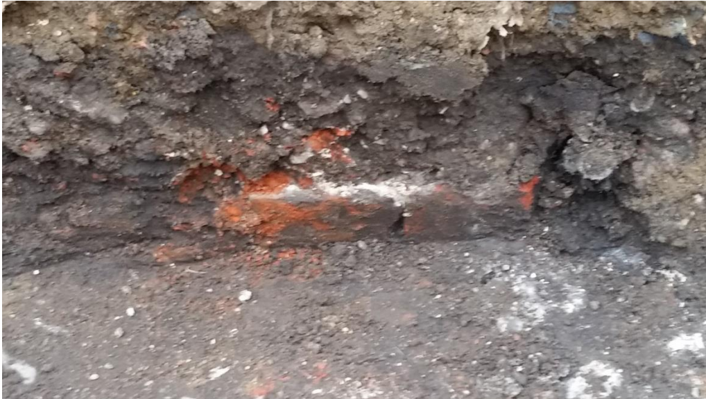
Plate 7. Part of brick wall 06 , looking east
