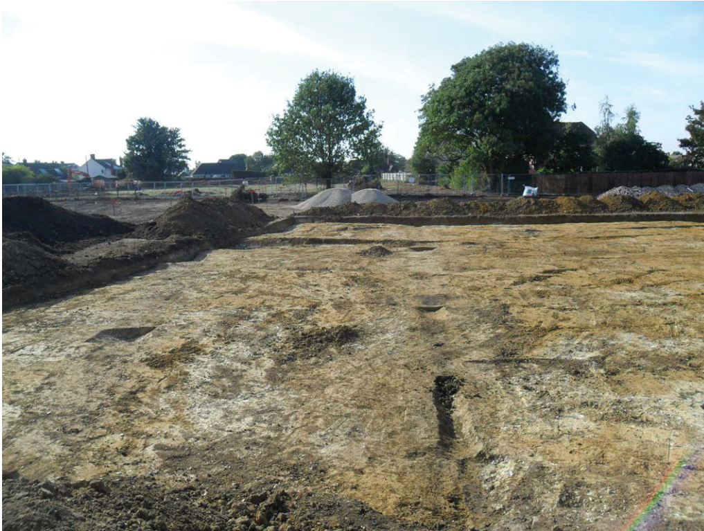
Plate 9. Excavation area with ditches MN[56] and MN[73], looking west
