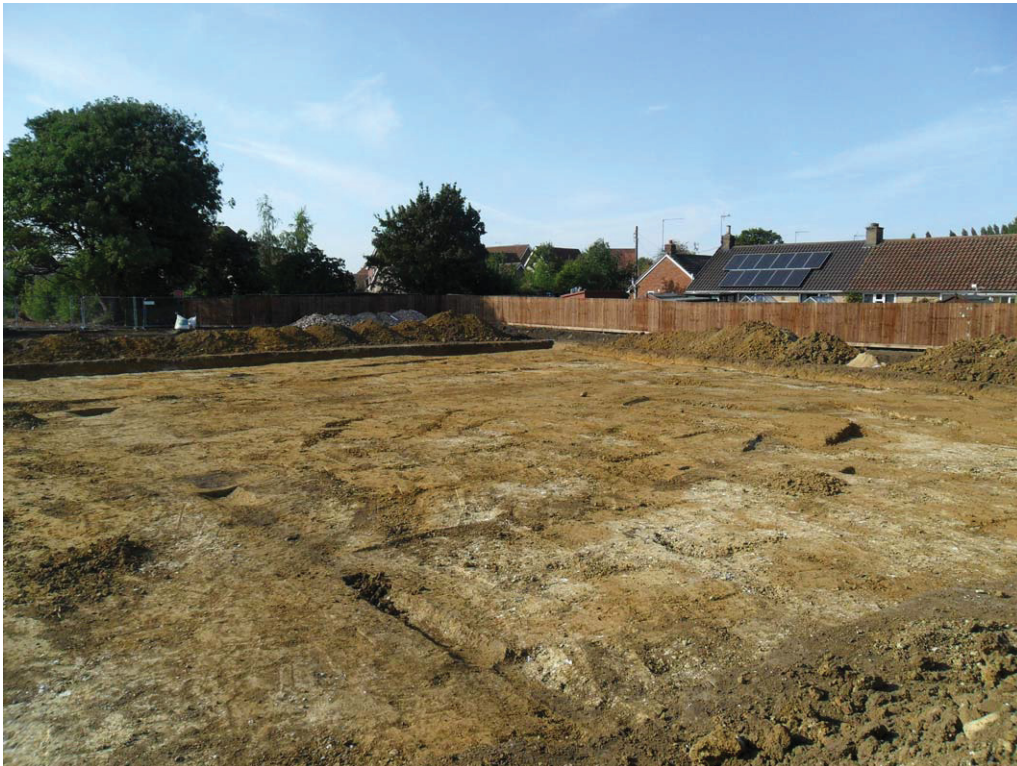
Plate 2. Excavation area, looking north-west
