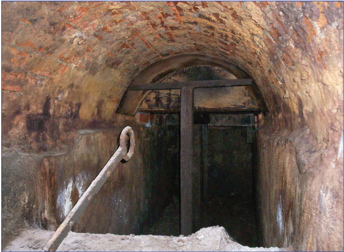
Plate 2 Arched brick culvert under King Street
