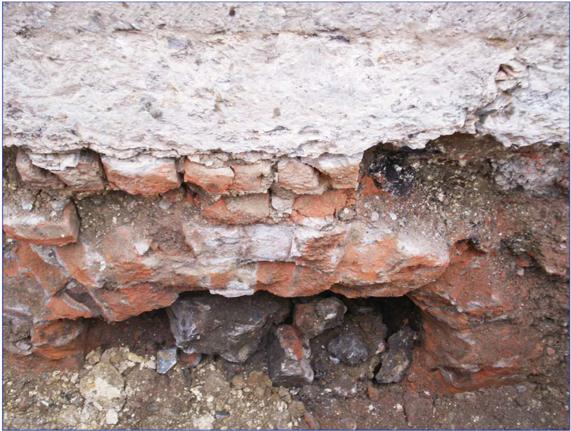
Plate 6 19th-century brick culvert
