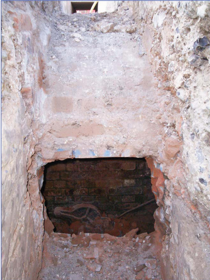
Plate 1 Brick culvert at junction of King Street and Carrow Hill
