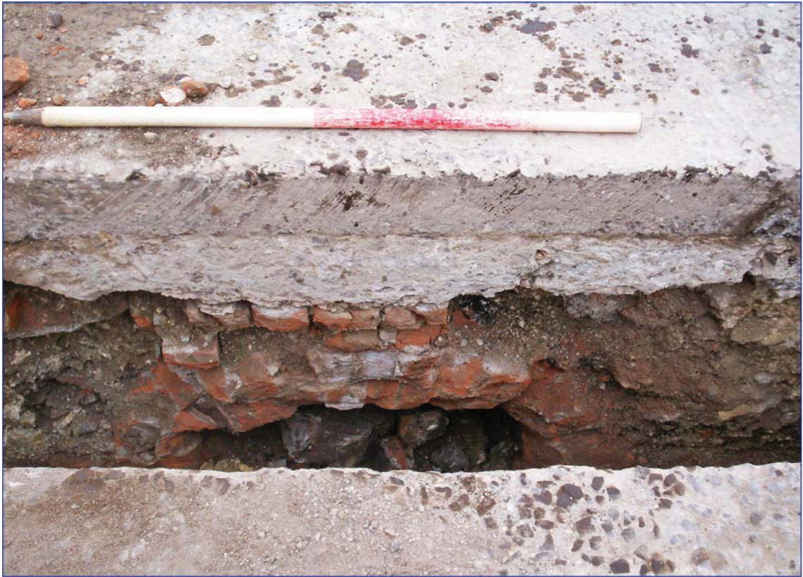
Plate 5 19th-century brick culvert
