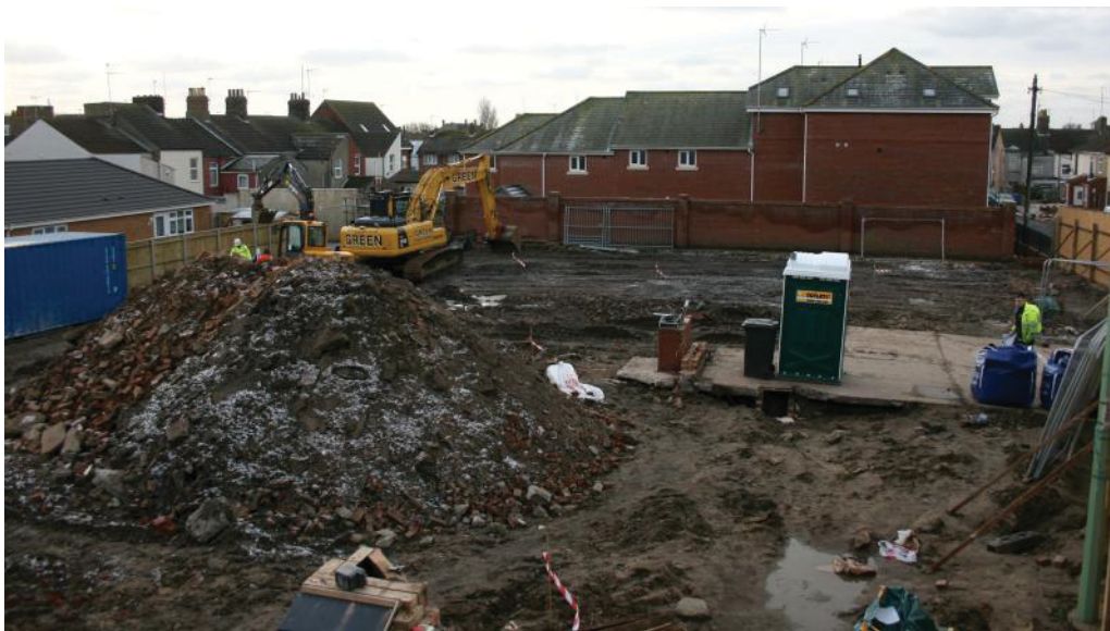
Plate 1. General view of site, looking south
