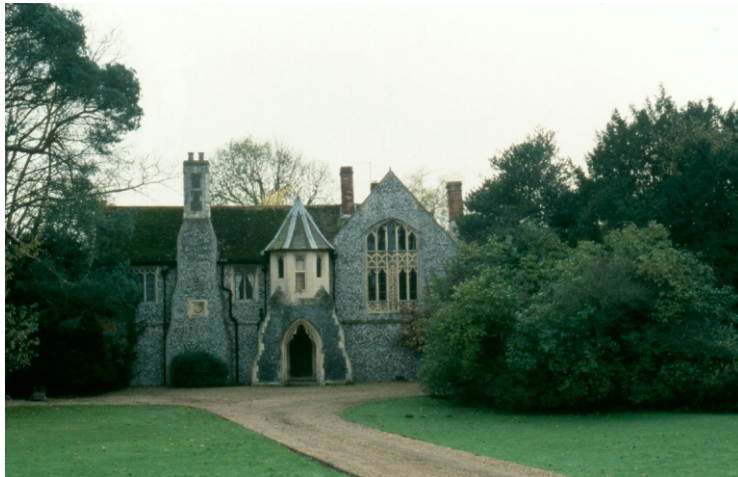
Plate 1. North facing facade of Rushford College. Looking south from churchyard.
