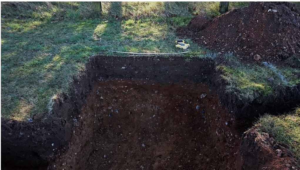
Plate 4. Soak-away 2, looking south
