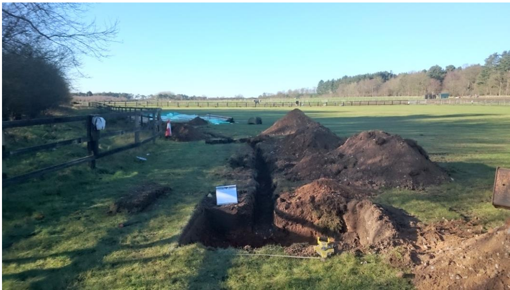
Plate 5. Pipe trench, looking west
