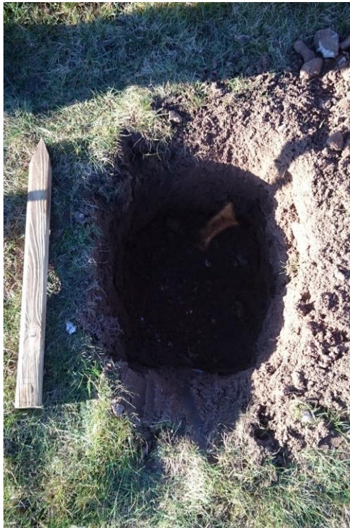
Plate 6. Example of a tree planting pit – alongside 0.60m stake
