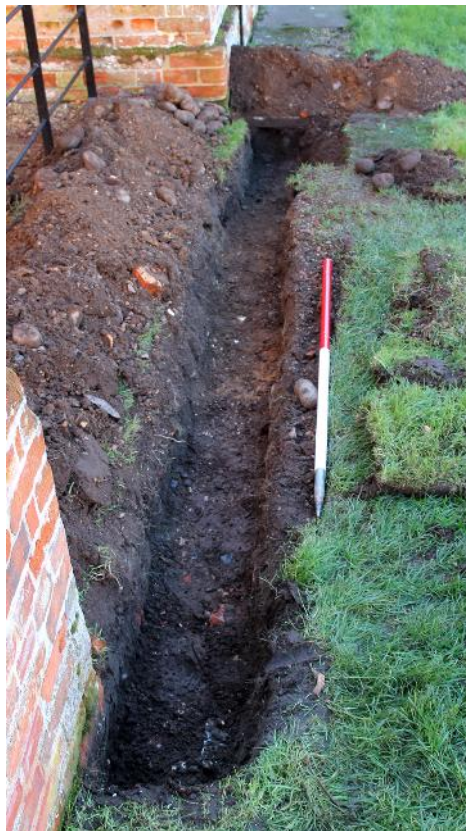
Plate 5. Excavation in service wing outbuilding courtyard. Looking south
