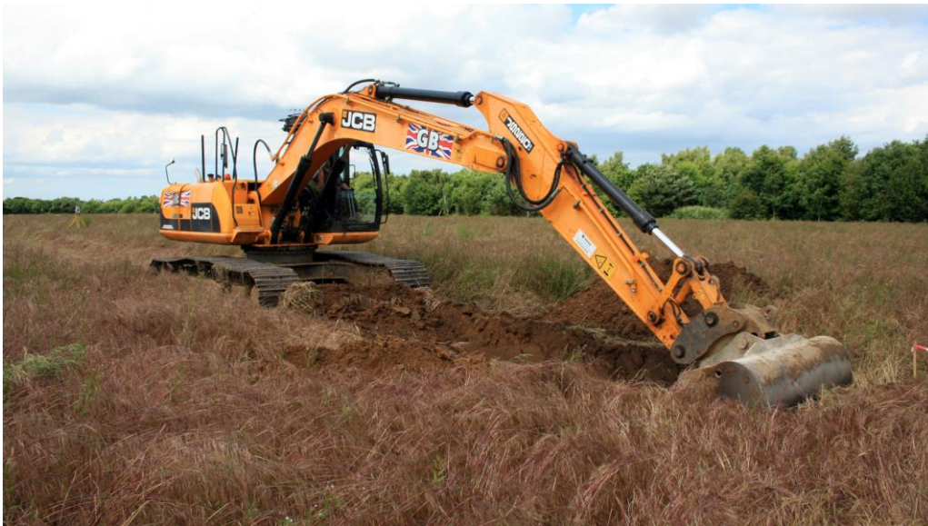
Plate 1. Machining looking northeast
