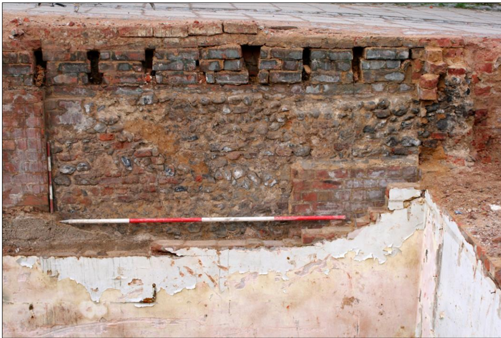
Plate 9. South facing elevation of wall 25
