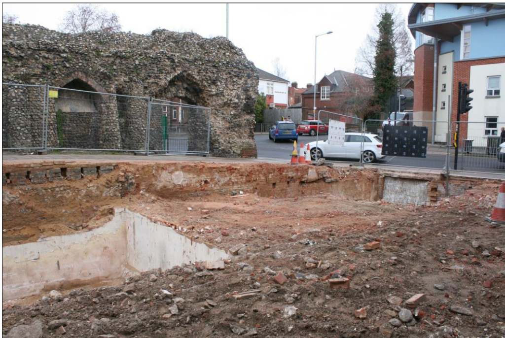
Plate 2. General view of work underway, looking north-east
