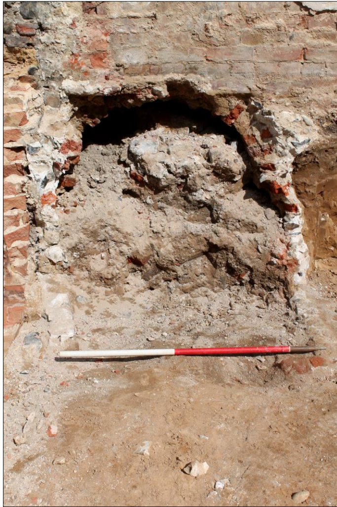
Plate 10. Vaulted cellar 51, looking north
