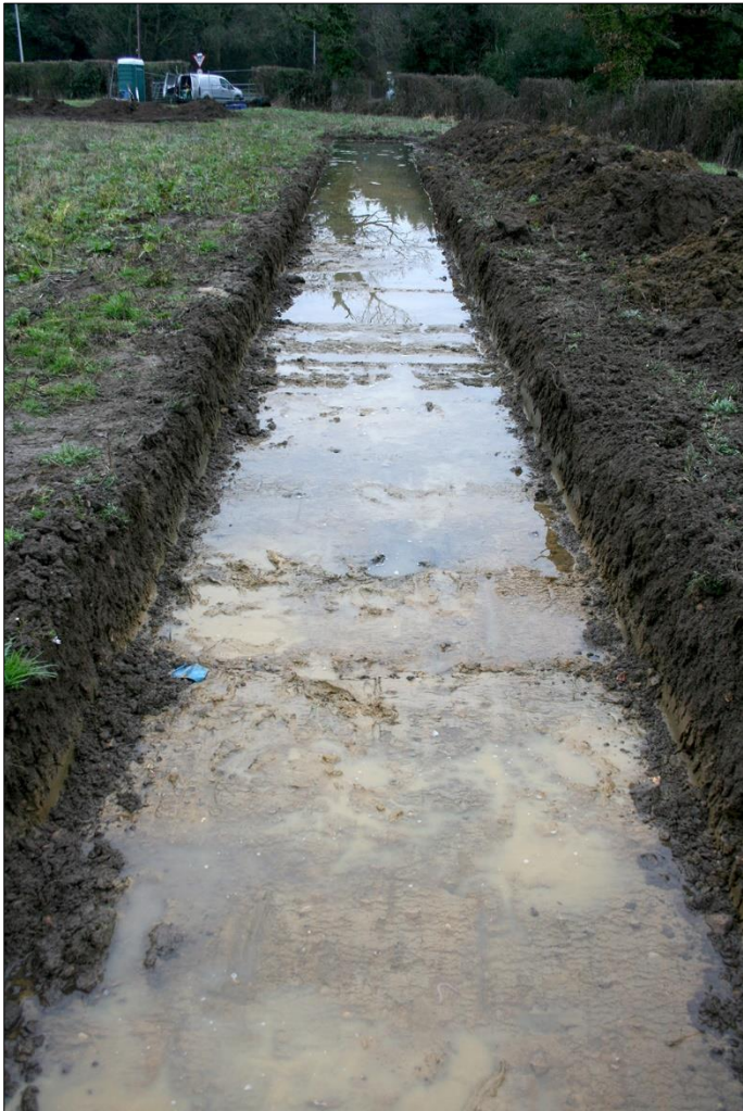
Plate 5. Trench 5, flood damage
