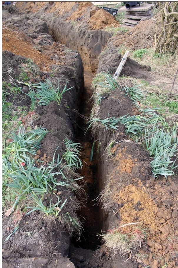
Plate 1. Monitored groundworks at Marble Hill Lodge North
