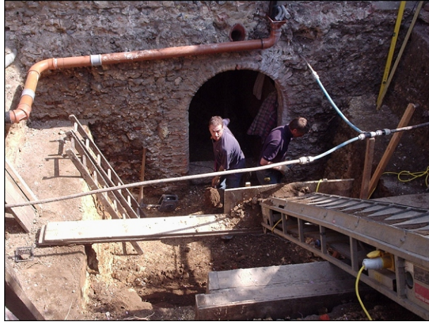
Plate 3 Working at base of conveyor belt
