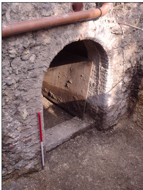
Plate 7 Entrance to the 17th century cellar
