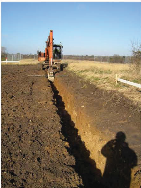
Plate 4 Foundations being dug in stripped area at far north of site
