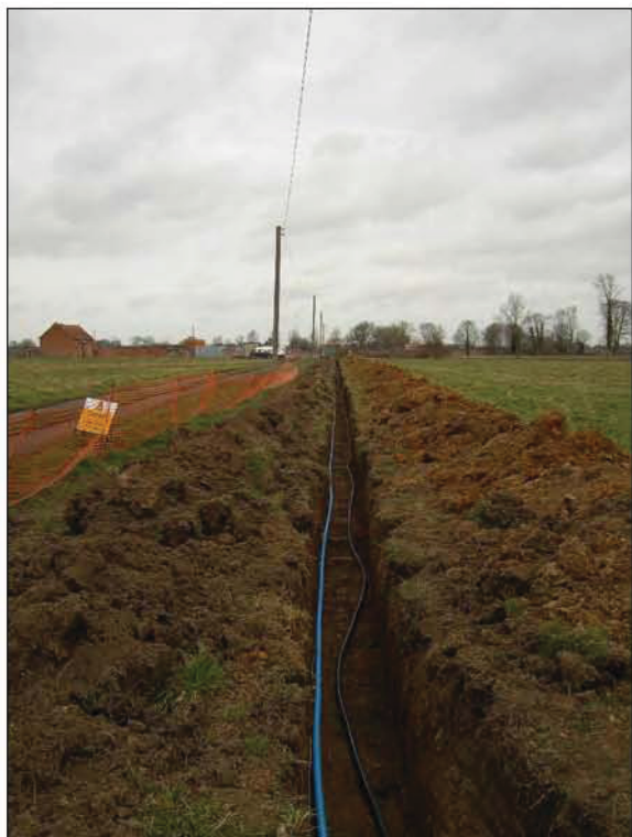
Plate 5 Excavated service trench, looking north towards the construction site
