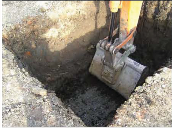
Plate 2 The deepest of the pilepits
