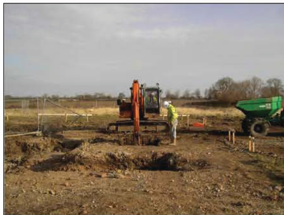
Plate 3 Excavation of pile pit
