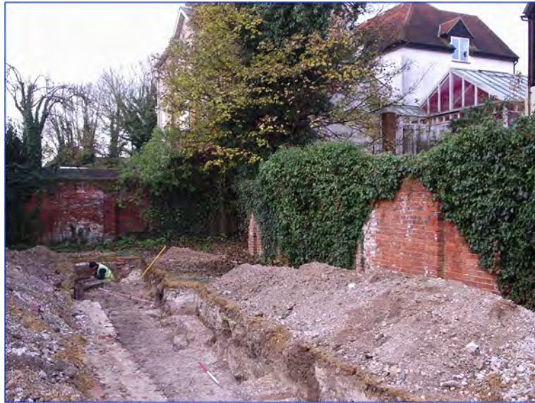
Plate 3 Excavation in progress, looking west
