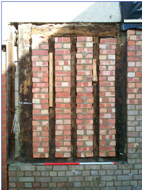
Plate 14 South wall of listed building, facing north
