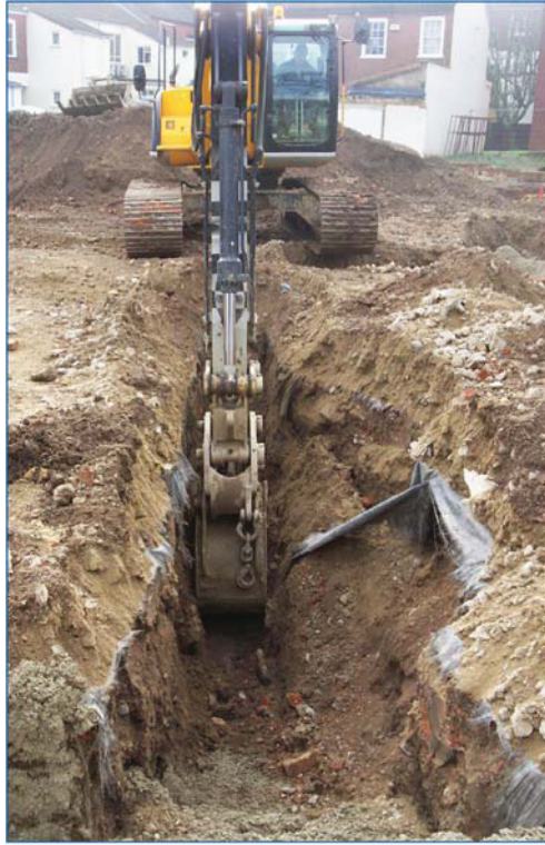
Plate 3 Thirty-tonne machine excavating foundations at the north of the site
