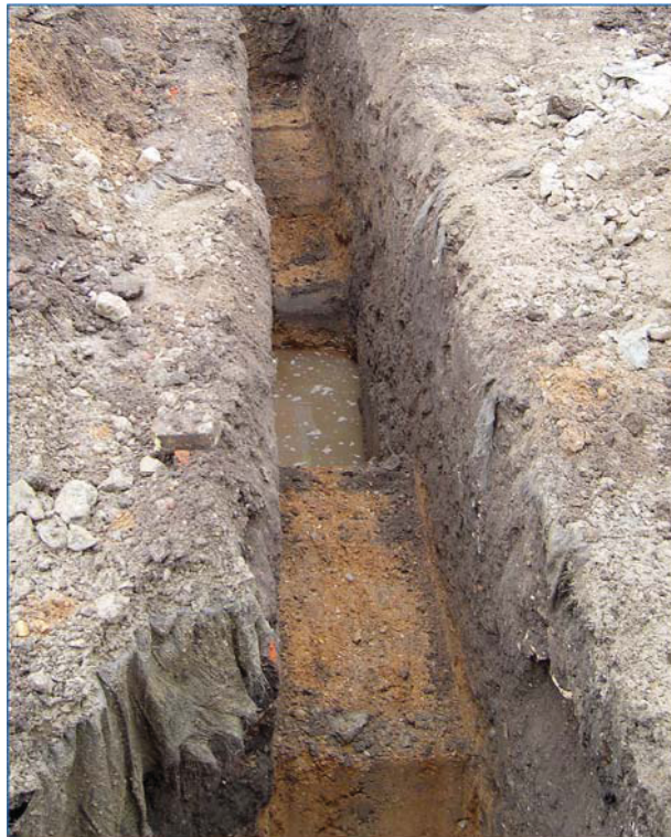
Plate 2 Pit visible in foundation trench in south-western corner of site
