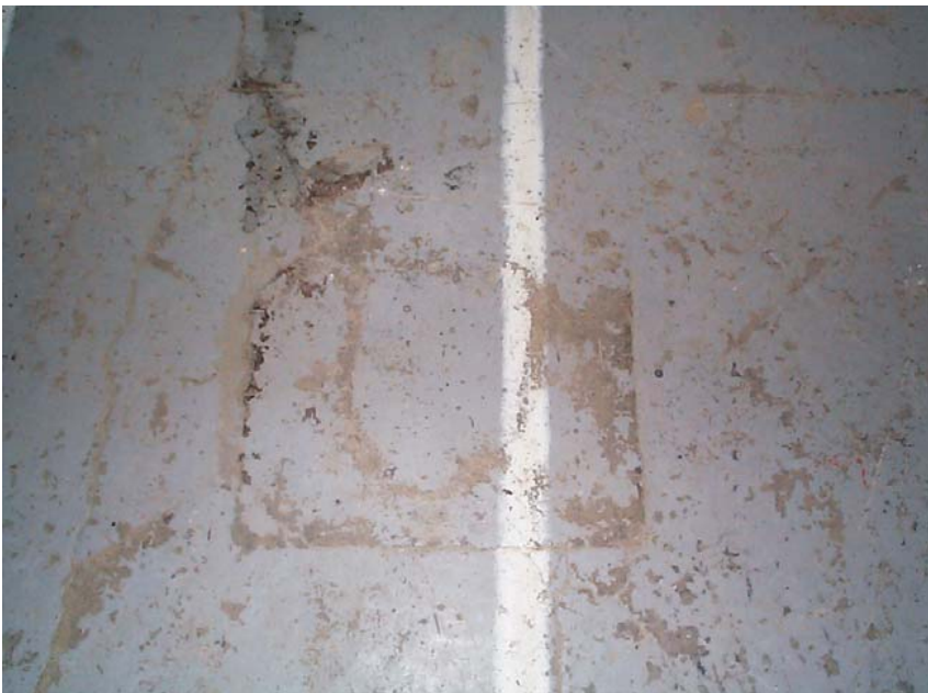
Plate 8 Stone base for Samson post preserved in later floor
