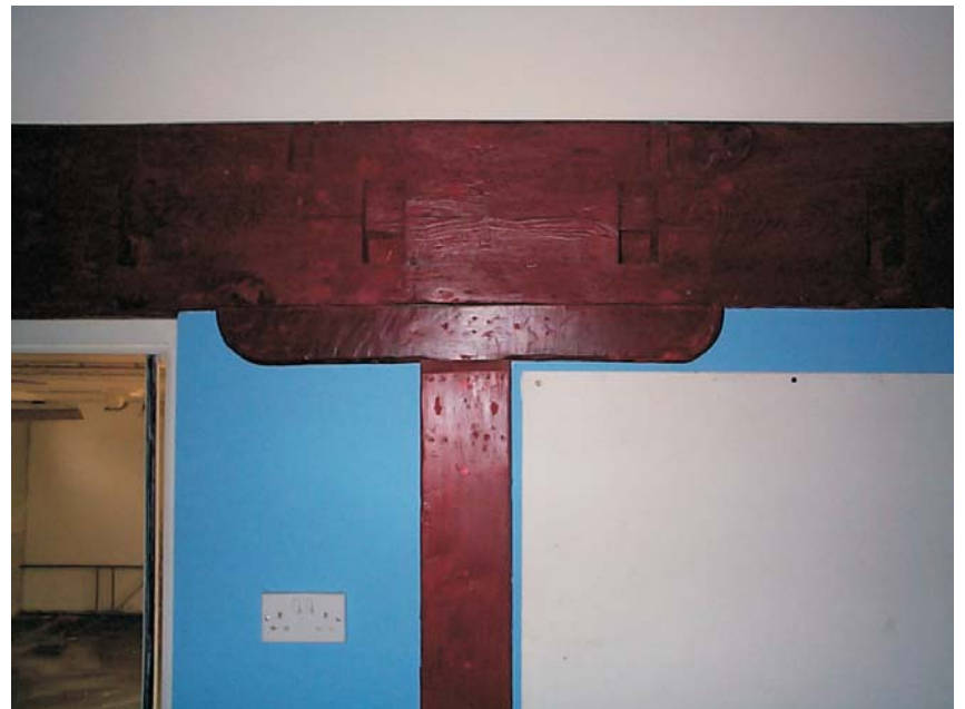
Plate 9 Tie-beam of south-west end truss showing joist mortises, pillow block and post
