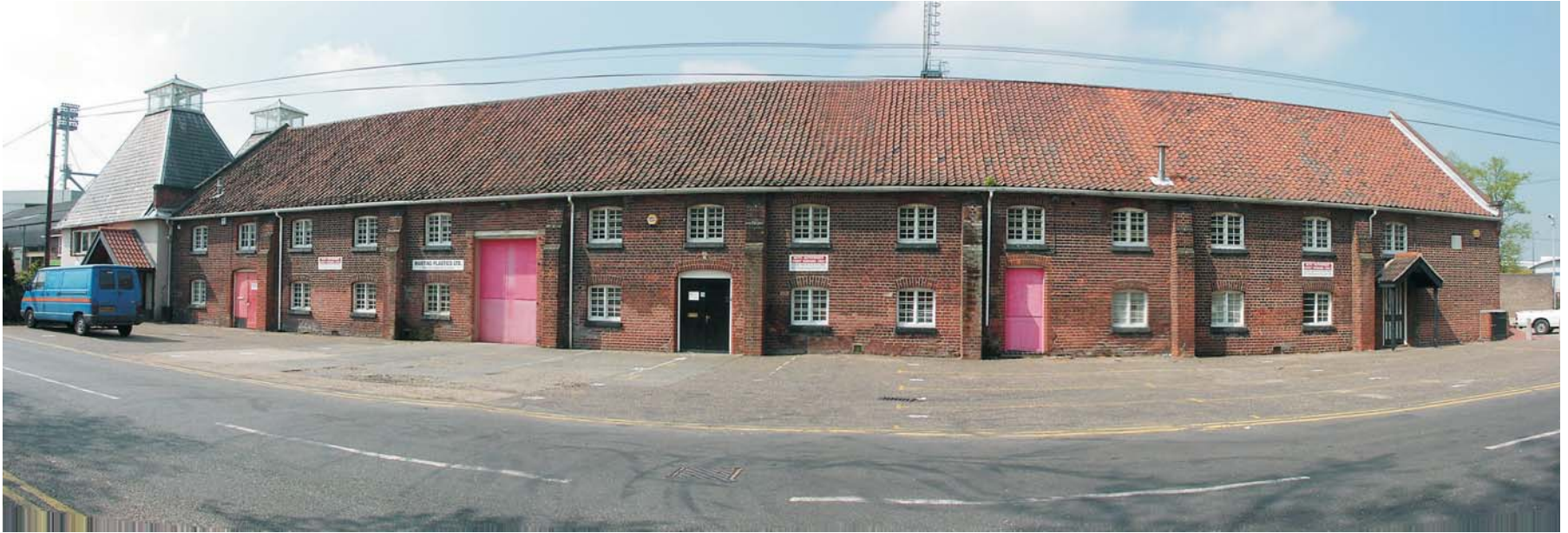
Plate 5 East-facing elevation of malthouse, by Robert Smith
