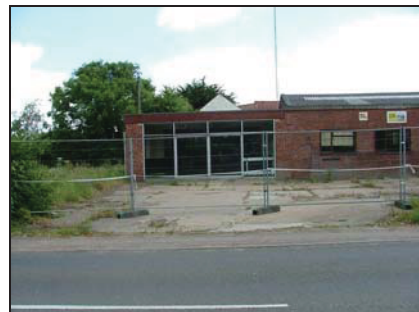
Plate 24. Part of west elevation of service station
