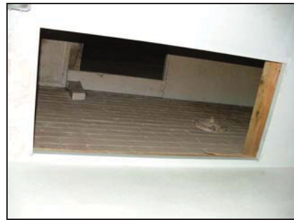
Plate 46. View of the wall between Buildings C and A
