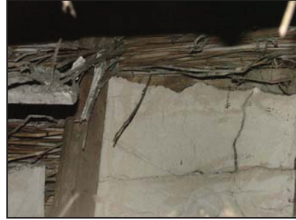
Plate 44. Roof space of Building B showing reeds/straw covered in plaster
