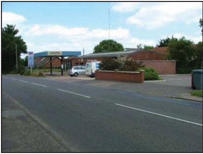
Plate 1. Salhouse Service Station on Mill Road as seen from the south
