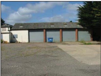
Plate 17. East-facing elevation of Building D
