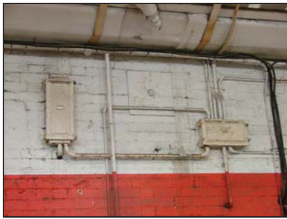
Plate 51. Square tie-plate, original east external wall of Building A
