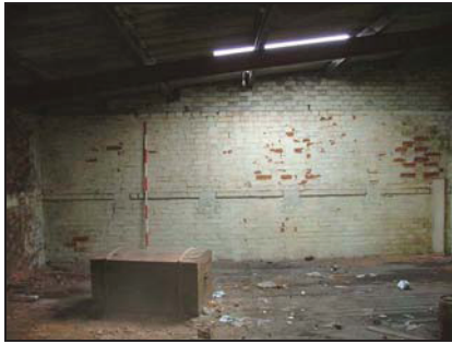
Plate 33. First floor, east wall at north end of Building A
