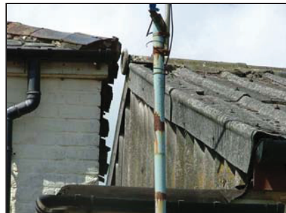
Plate 18. Detail of the circular feature on south elevation of Building D
