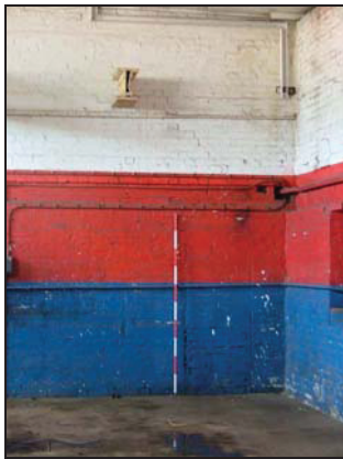
Plate 27. Blocked doorway in northern cross-wall, interior of Building A
