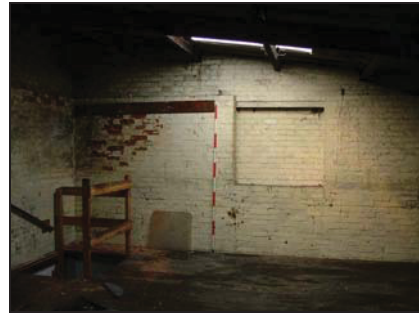
Plate 34. First floor, north end of Building A
