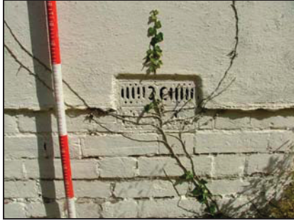
Plate 7. Decorative ventilation grilles in south elevation of Building A
