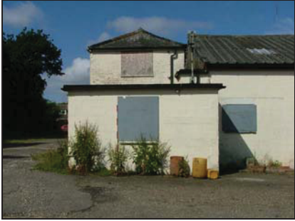
Plate 13. East-facing elevation of Building B
