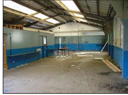
Plate 56. Interior of Building E which faces Mill Road, view looking north
