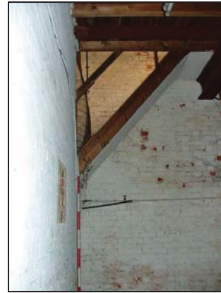
Plate 30. Redundant stairs in north-west corner of Building A
