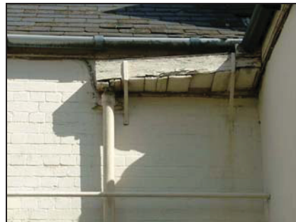
Plate 16. Rainwater hopper, south elevation of Building C
