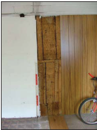
Plate 45. North internal wall, first floor, Building B
