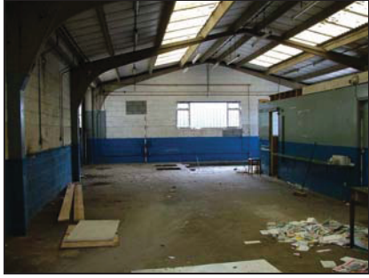
Plate 55. Interior of Building E which faces Mill Road
