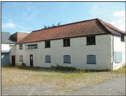
Plate 3. West elevation of buildings to the rear of modern service station
