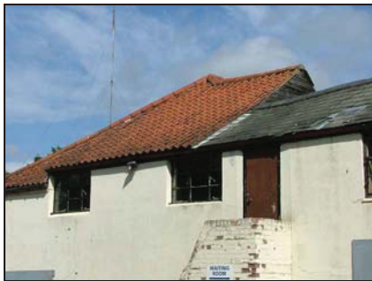
Plate 9. Change in roof lines and materials between Buildings A and B
