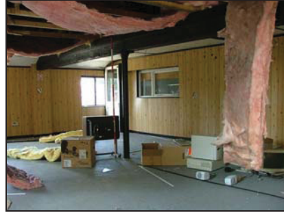
Plate 38. South end of Building A, first floor
