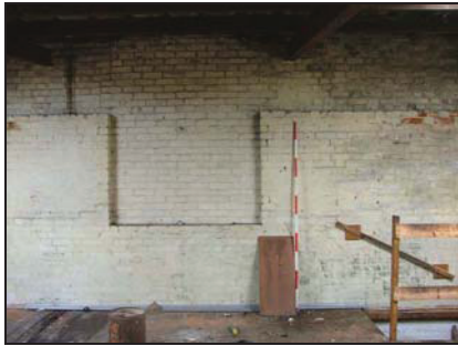
Plate 35. First floor, north end of Building A, south wall
