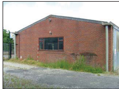
Plate 22. South elevation of former service station
