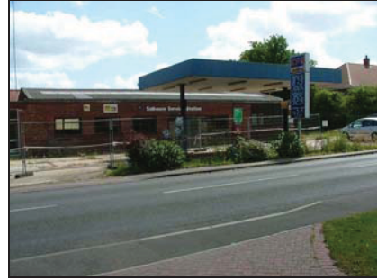
Plate 20. West elevation of Building E fronting Mill Road
