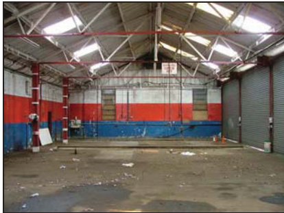
Plate 47. View looking north of the interior of Building D
