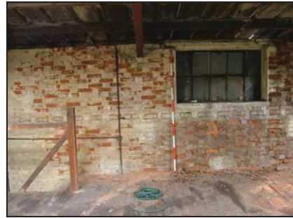
Plate 36. First floor, north end of Building A, north wall
