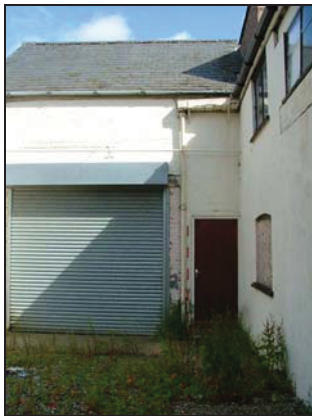
Plate 15. South-facing elevation of Building C
