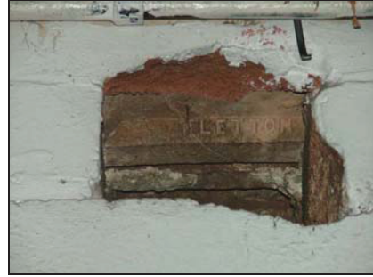
Plate 32. 'Fletton' brick visible in northern interior cross-wall in Building A
