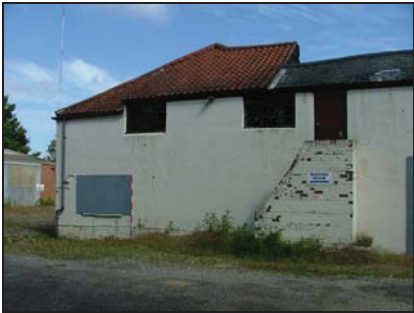
Plate 5. South elevation of Building A
