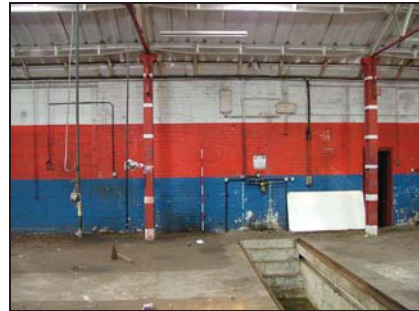
Plate 48. West wall of Building D showing blocked door
