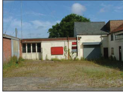
Plate 14. View looking north showing Building C
