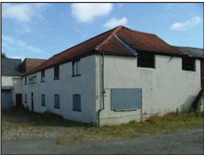
Plate 4. South elevation of Building A
