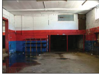
Plate 26. View looking south of interior of Building A
