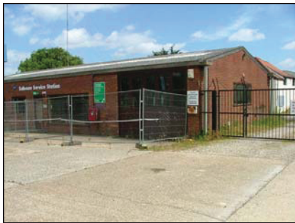
Plate 21. Main service station building fronting Mill Road
