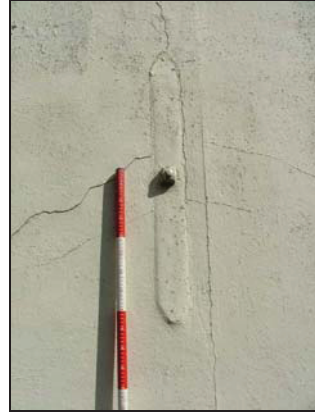
Plate 8. Metal wall tie, south wall of Building A
