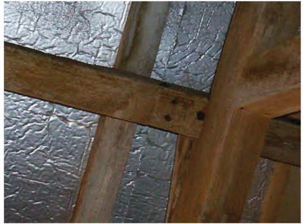
Plate 8. Carpenter's makings on west truss, Building A
