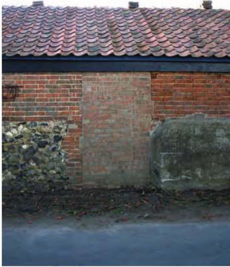
Plate 7. Blocked doorway in eastern elevation of Building B
