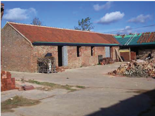
Plate 3. South-facing elevation of Building A, looking north-east
