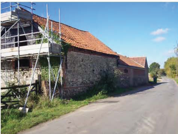
Plate 5. East-facing elevation of Building C, looking north
