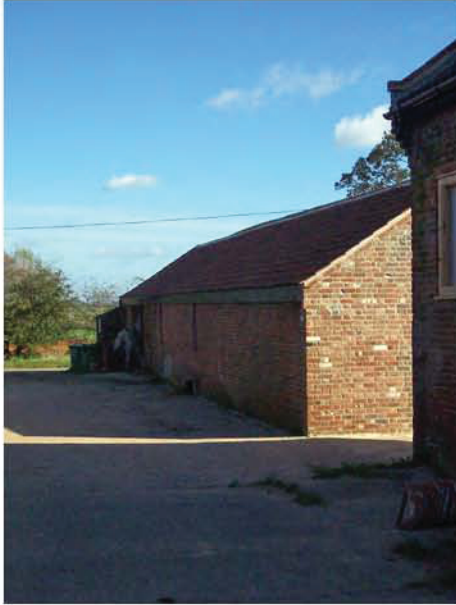
Plate 1. North-facing elevation of Building A, looking east
