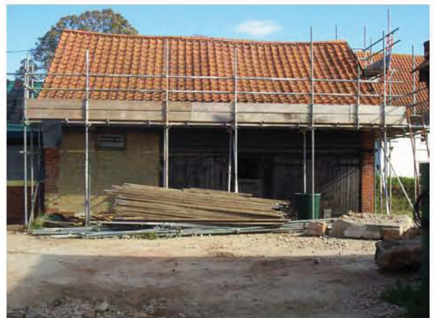
Plate 6. West-facing elevation of Building C, looking east
