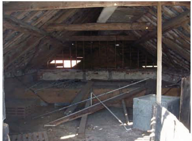
Plate 10. Internal view of Building C loft, looking north
