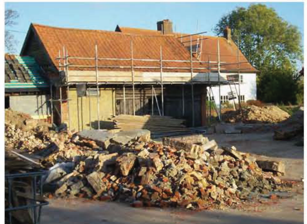
Plate 4. West-facing elevation of Building C
