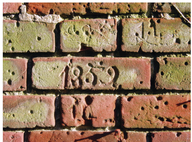
Plate 6. Inscription on gable wall of Building C
