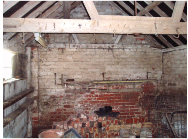
Plate 8. Area worn smooth and concave on gable wall of Building C, facing west
