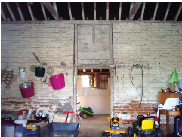
Plate 3. Western doorway of Building A, from interior
