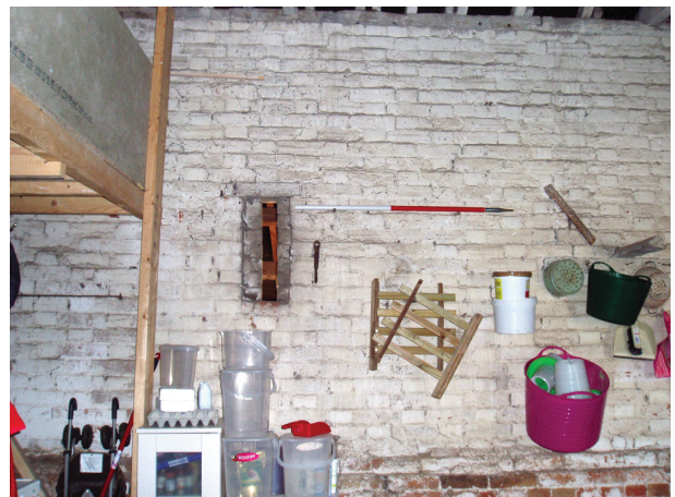
Plate 4. Ventilation slot on west wall of Building A, interior. Scale 1m
