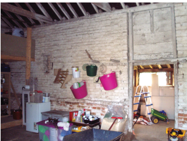
Plate 5. Interior of west wall showing plinth in Building A, looking south-west
