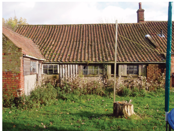
Plate 9. Building D, facing east
