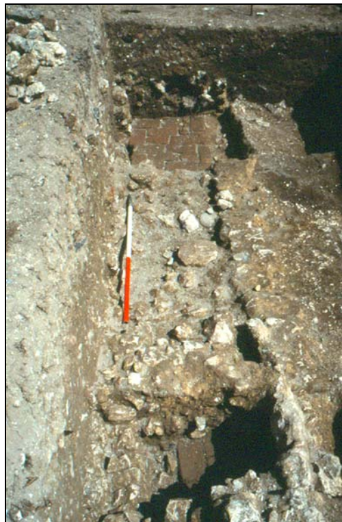
Plate 3. Excavated Culvert 31 showing partly collapsed roof.
